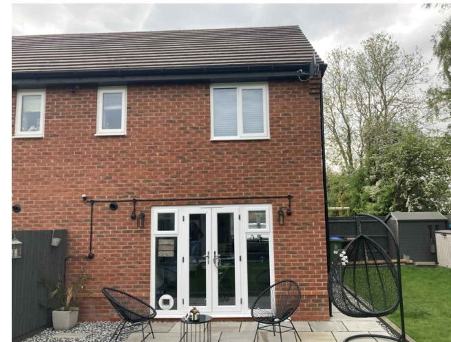
Photo 1: Existing rear elevation
