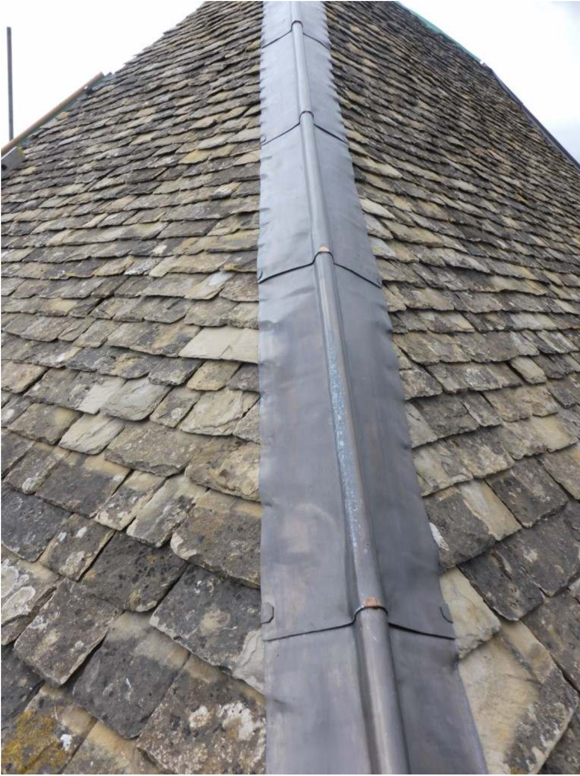
Completed lead hip
