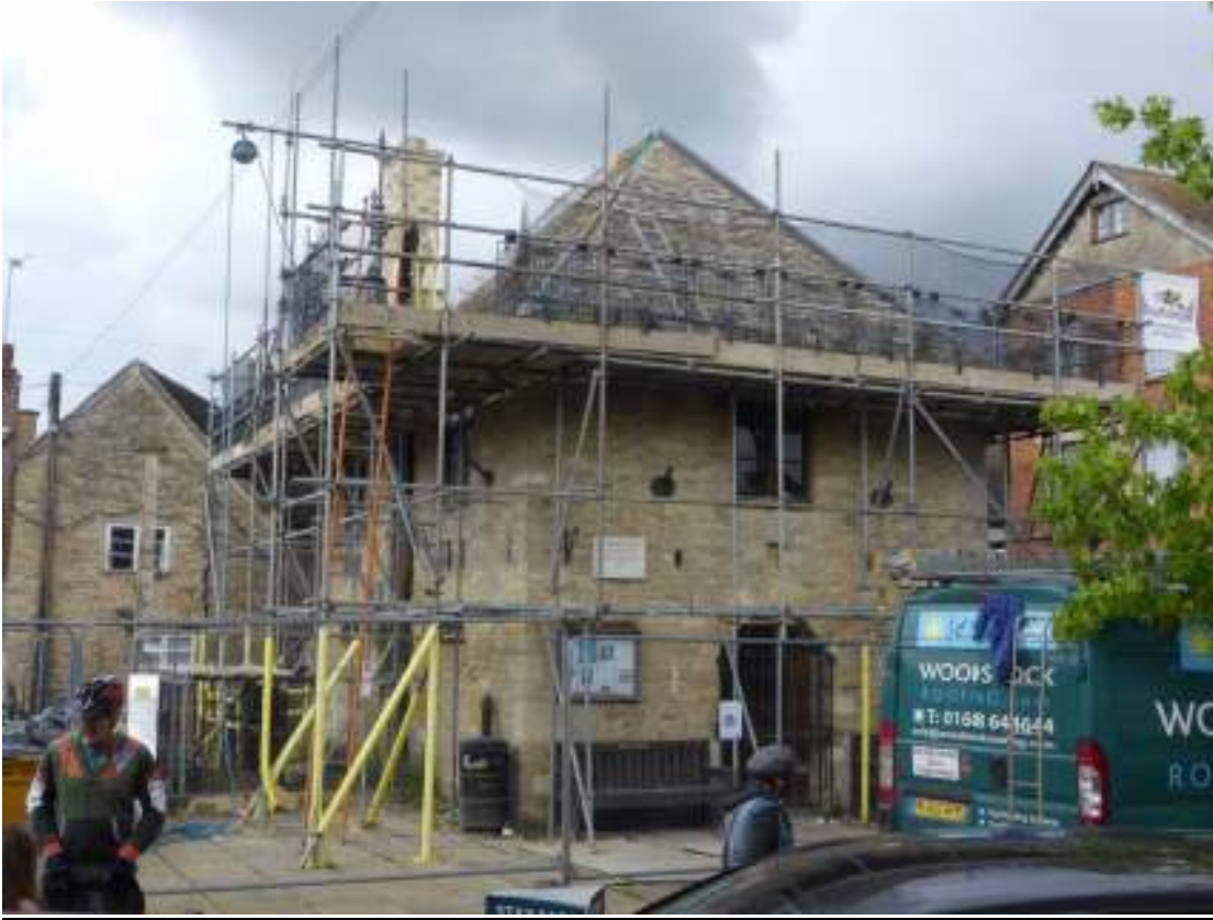
General view of the Bartholomew Building, presently scaffolded
