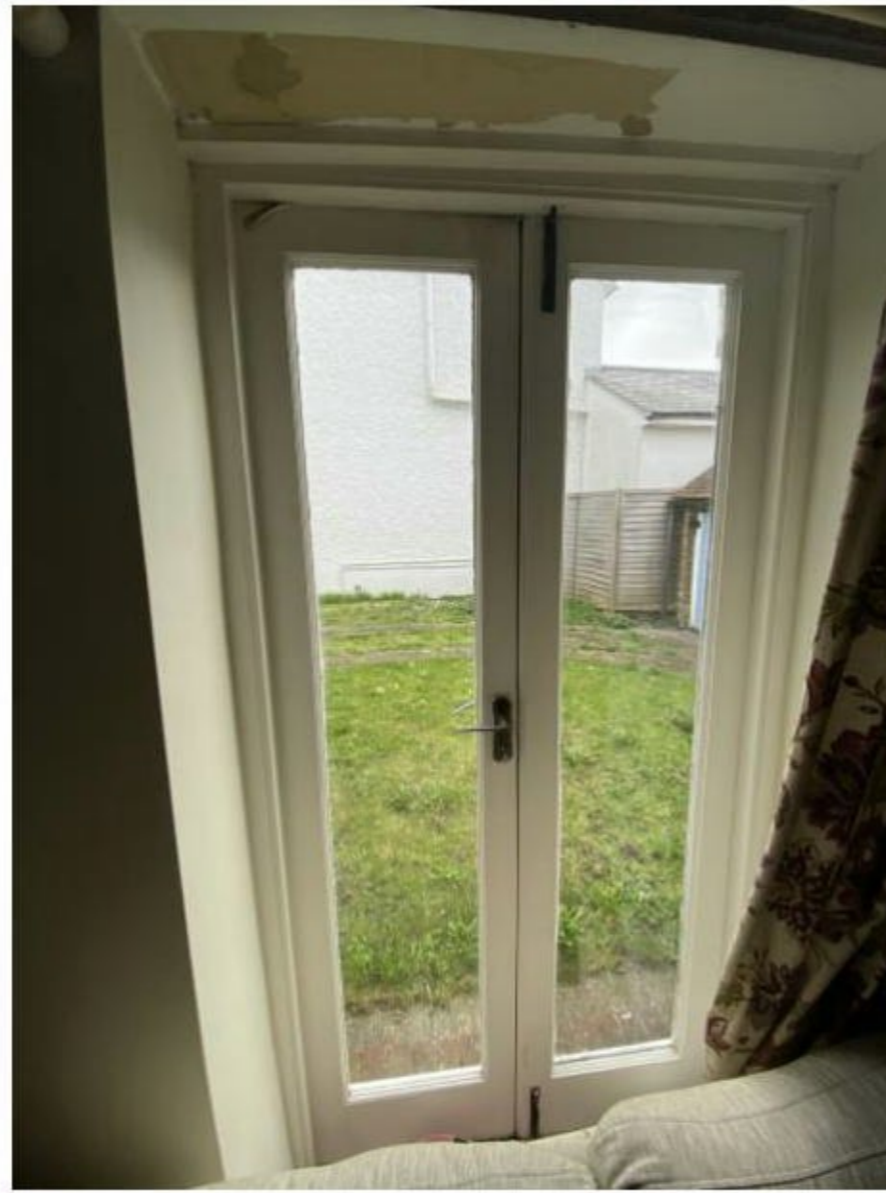
Existing doors retained
