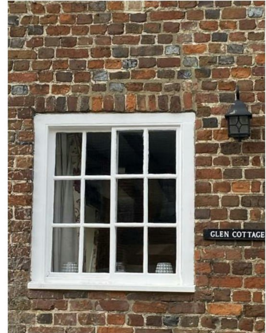
Existing timber window
