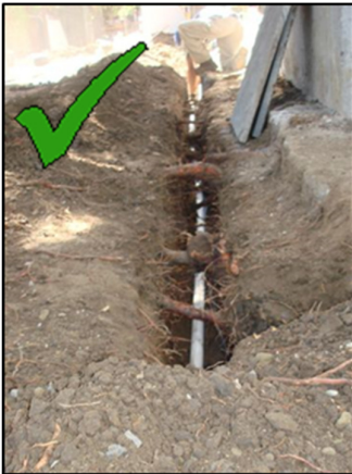
Significant roots retained
