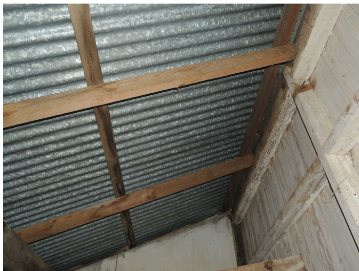
Photo 9: The roof lacked potential roosting places for bats
