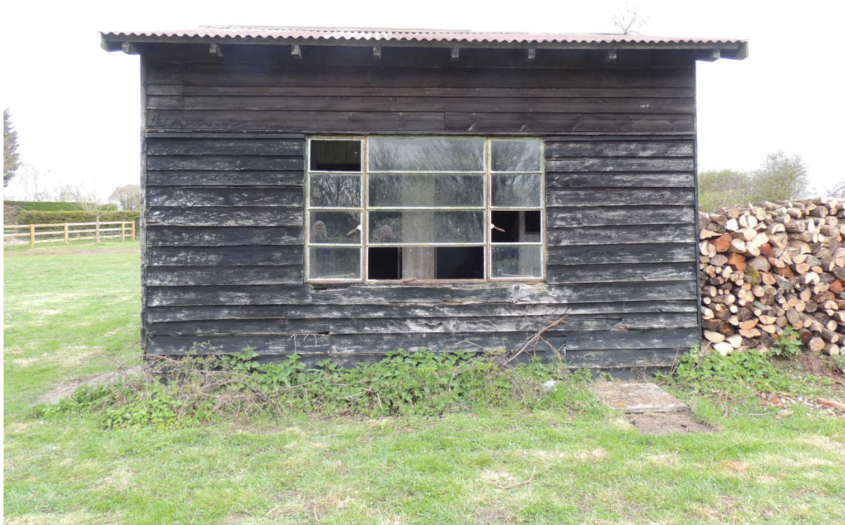
Photo 1: Southern elevation. Note large window
