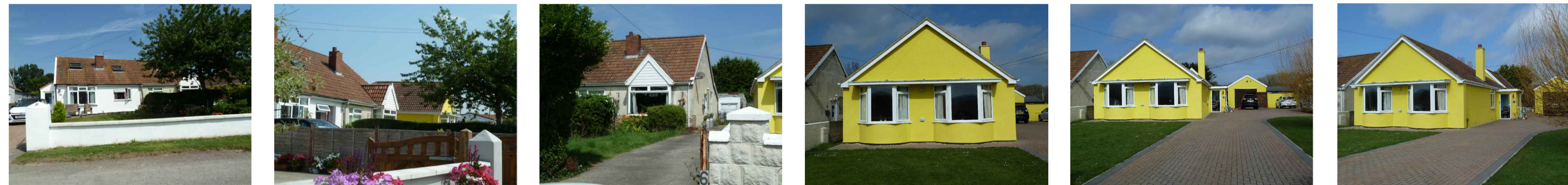
Views of the existing bungalows at 5 and 6 Hutton Moor Lane
