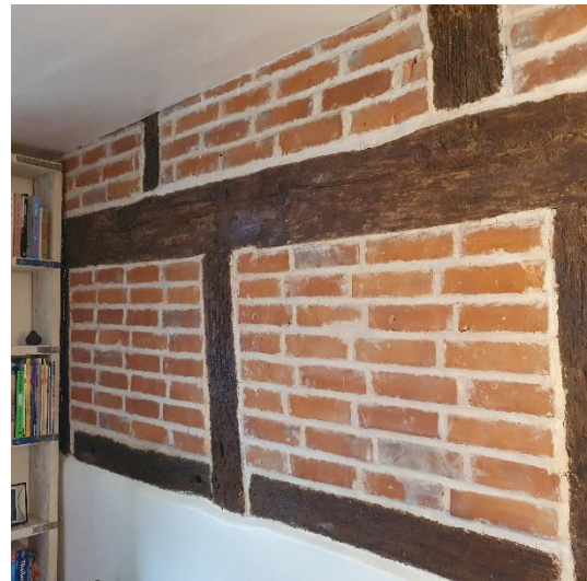
Beams to side wall
