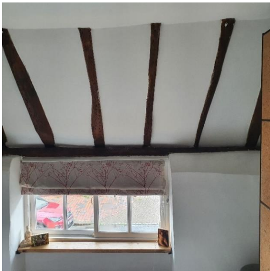
Rafters in Bedroom 1
