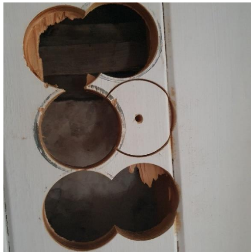
Holes in kitchen, lathe in top section, mortar below
