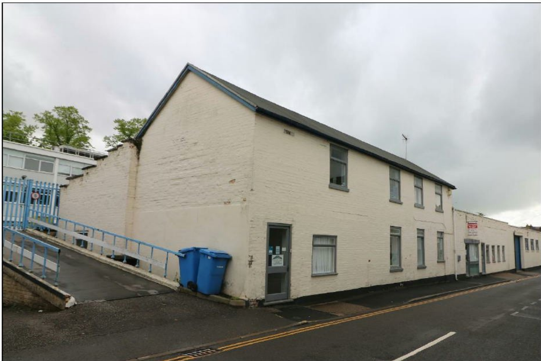
Figure 14 Remodelled 19 th century outbuildings with possible ghost mark of earlier gable
