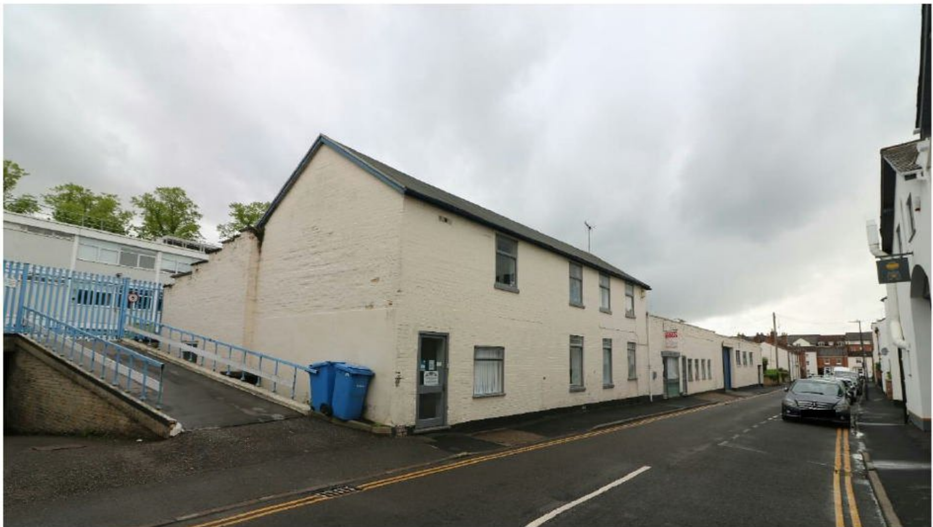
Figure 7 Late 18 th century outbuilding incorporated into mid-20 th century linear range
