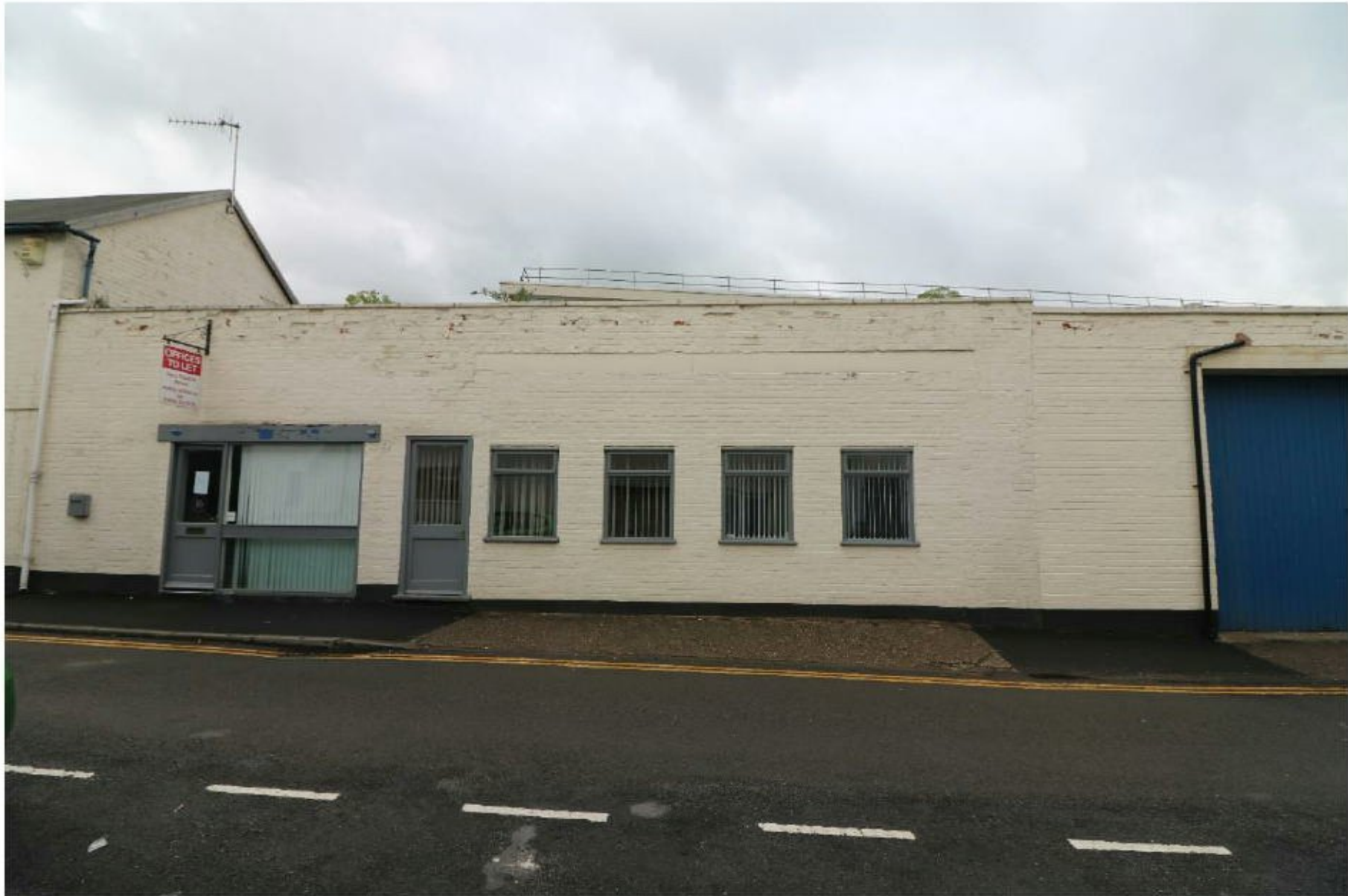
Figure 15 Wide lintel and window inserts to mid-20 th century industrial building over the west of the Site
