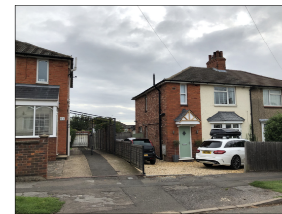
Photo of the front of Property
