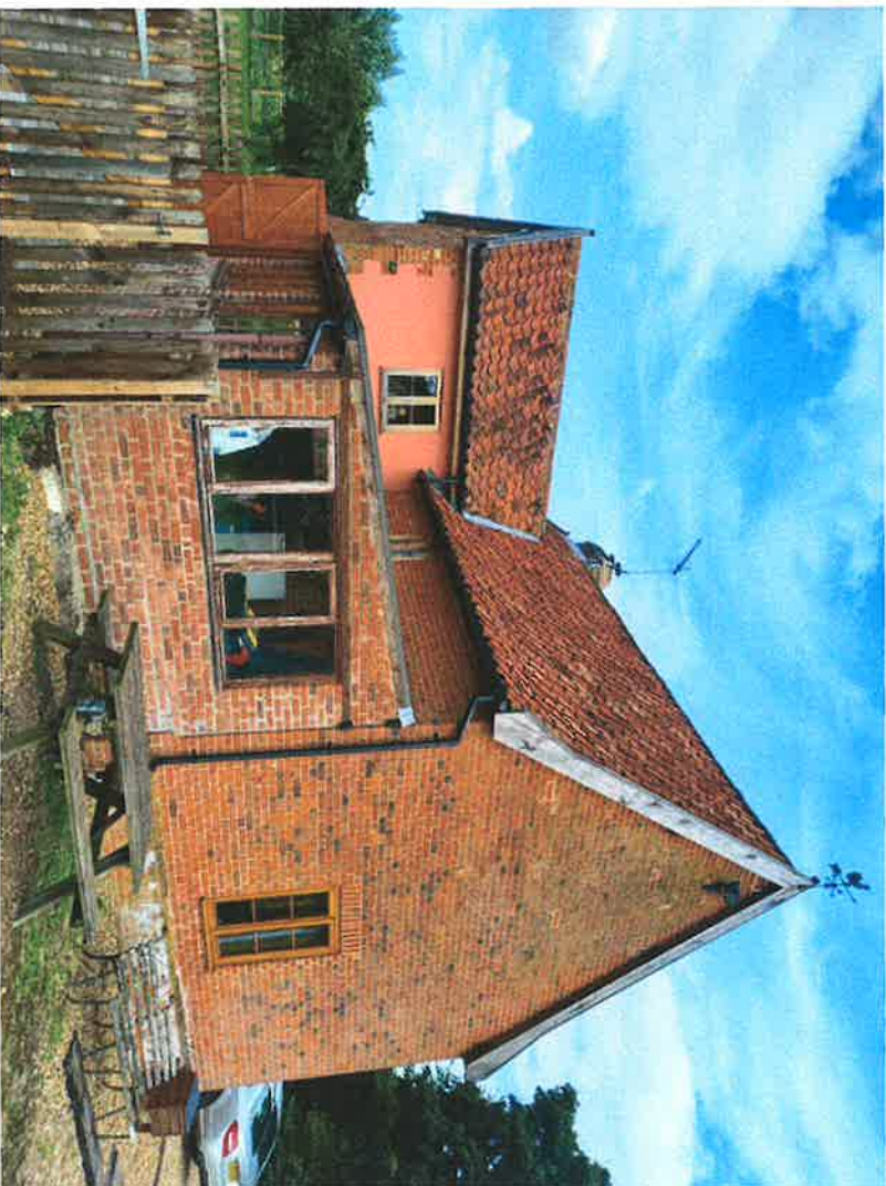
Side view of the property showing poor detailing of the conservatory and use of standard joinery combined to make a larger side window frame.
