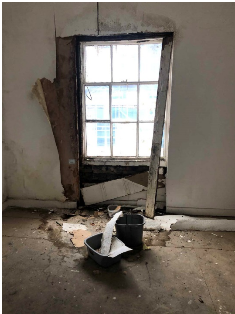
Existing W26 to be replaced
