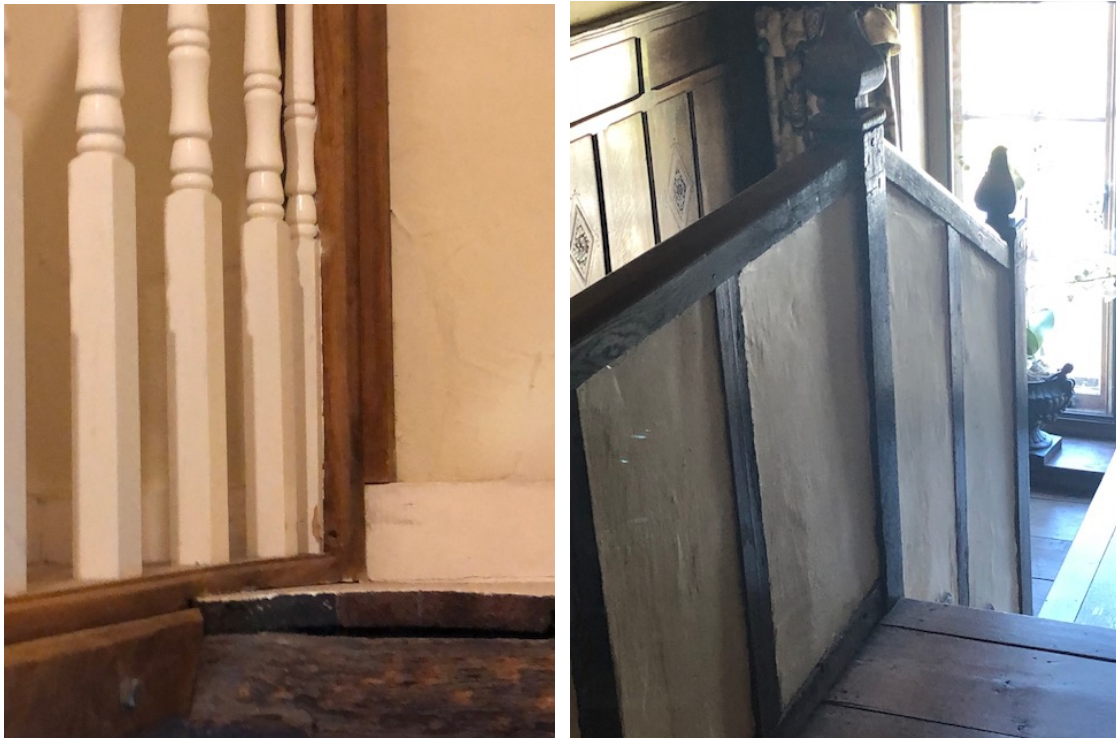
Plates 7 and 8. The modern spindles (left) would be replaced by a more appropriate style, such as those on the main staircase (right).
