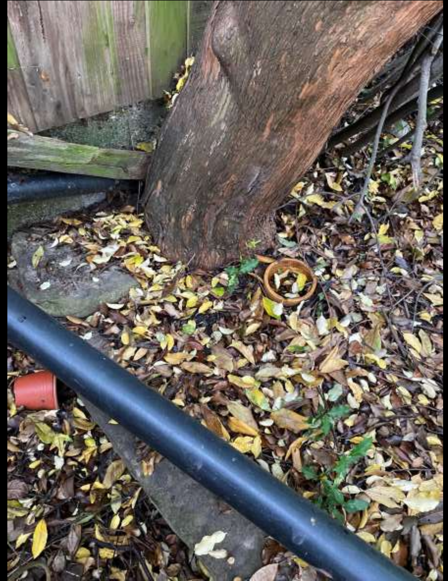
Detail of tree trunk in relation to rainwater pipe and fence.
