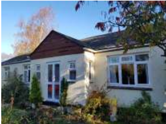
Plate 1: West elevation showing area of timber cladding where bats have been recorded roosting
