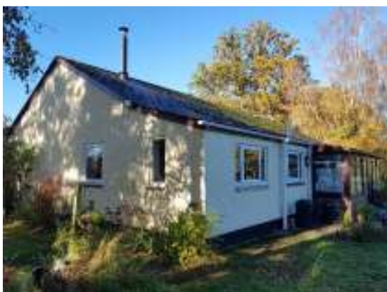
Plate 5: South and east elevations
