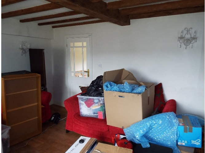
Figure 33. Ph 123. South wall of G4
