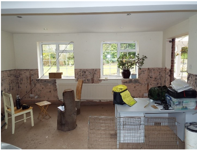
Figure 26. Ph 89. West wall, GF2
