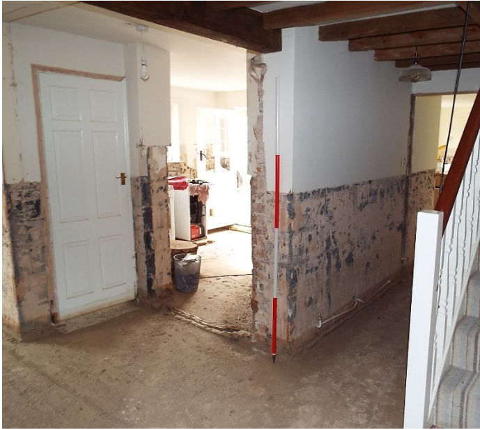
Figure 40. Ph 75. Ground floor hallway
