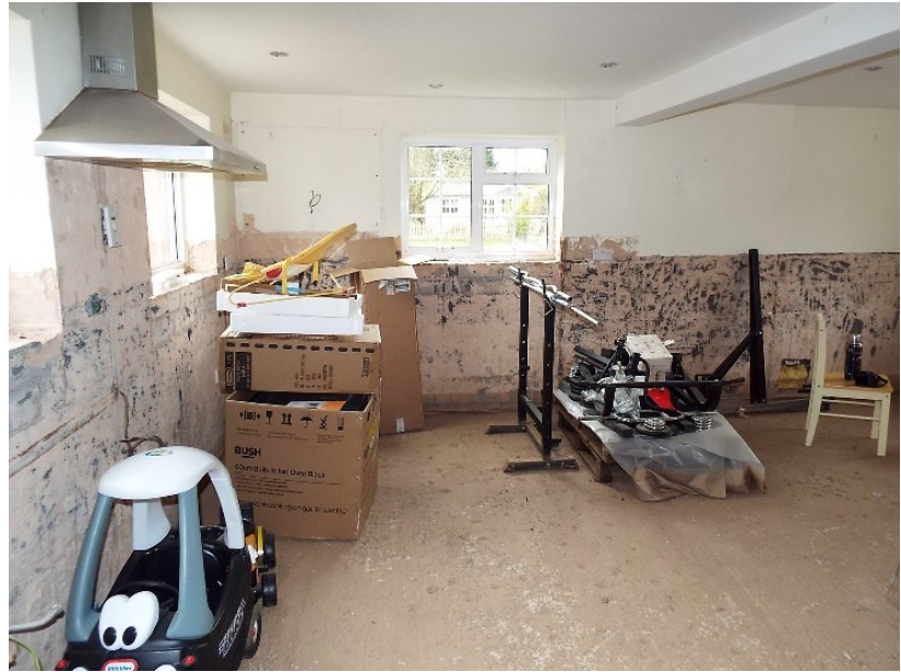
Figure 25. Ph 87. South and east walls, GF2
