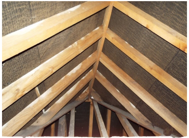
Figure 58. Ph 244. Roof structure facing east
