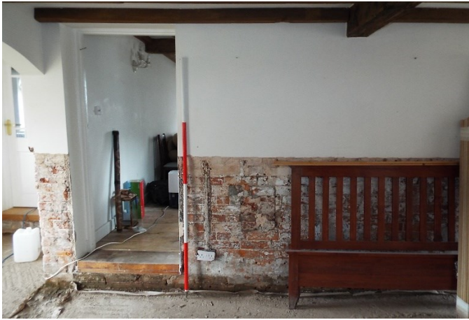
Figure 38. Ph 151. South wall of G5
