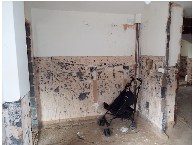
Figure 23. Ph 82. West wall GF1
