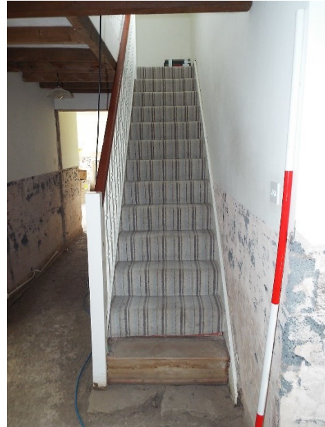
Figure 41. Ph 74. Stairs to first floor
