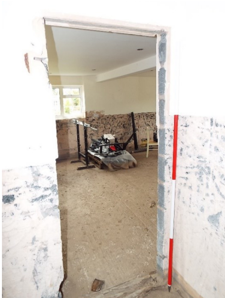
Figure 24. Ph 86. Doorway of South wall, GF1
