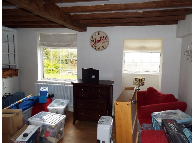
Figure 31. Ph 119. North wall of G4
