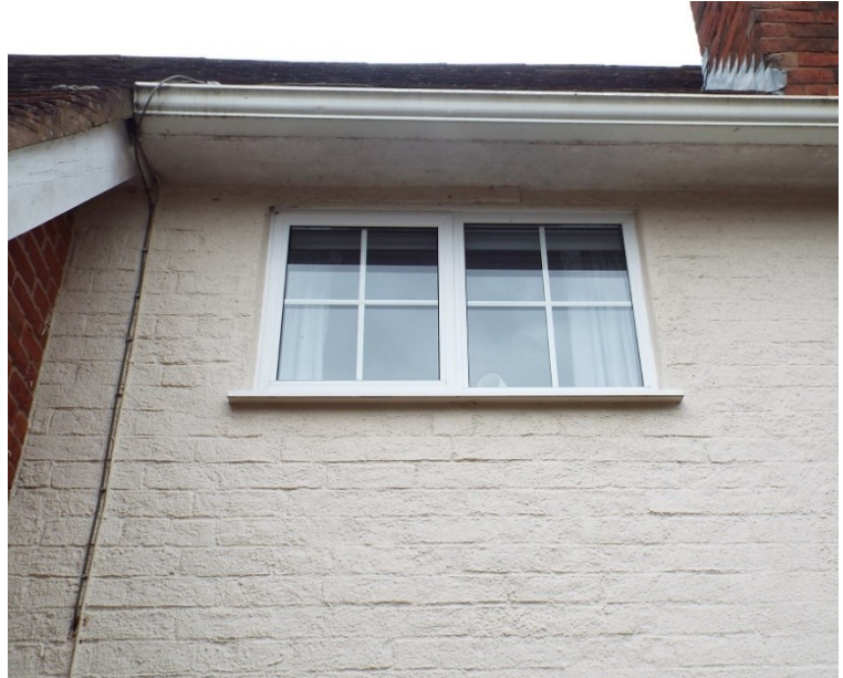
Figure 18. Ph 67. First floor window
