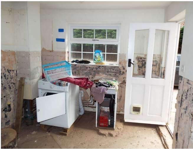
Figure 22. Ph 81. East wall GF1
