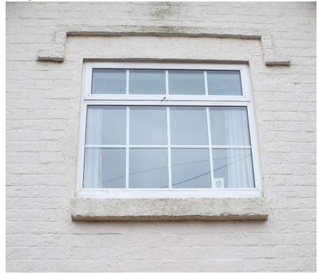
Figure 12. Ph 13. First floor window
