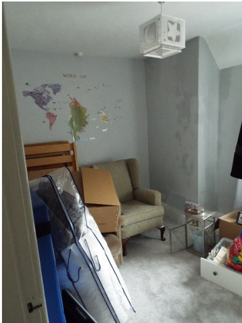
Figure 45. Ph 181. FF2 north and west walls
