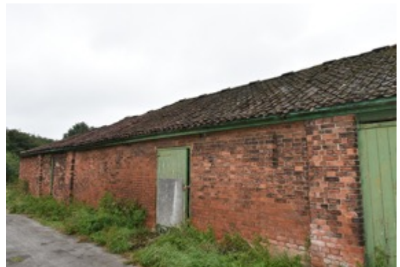
Image 4: East facing side aspect of B2
