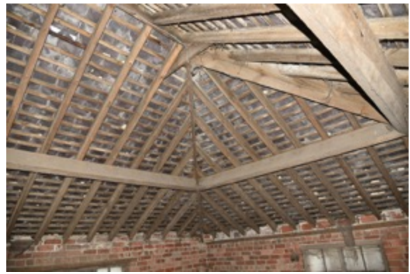
Image 2: Internal roof structure of B1
