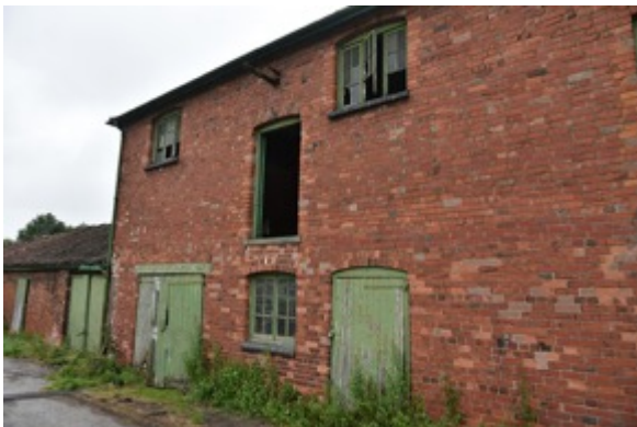
Image 1: East facing side aspect of B1
