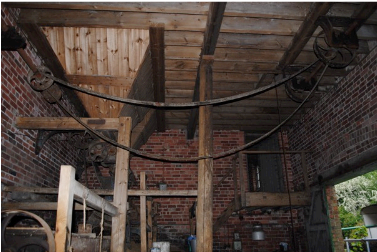
Plate 10: Plot 2, internal ground floor, as viewed looking west.
