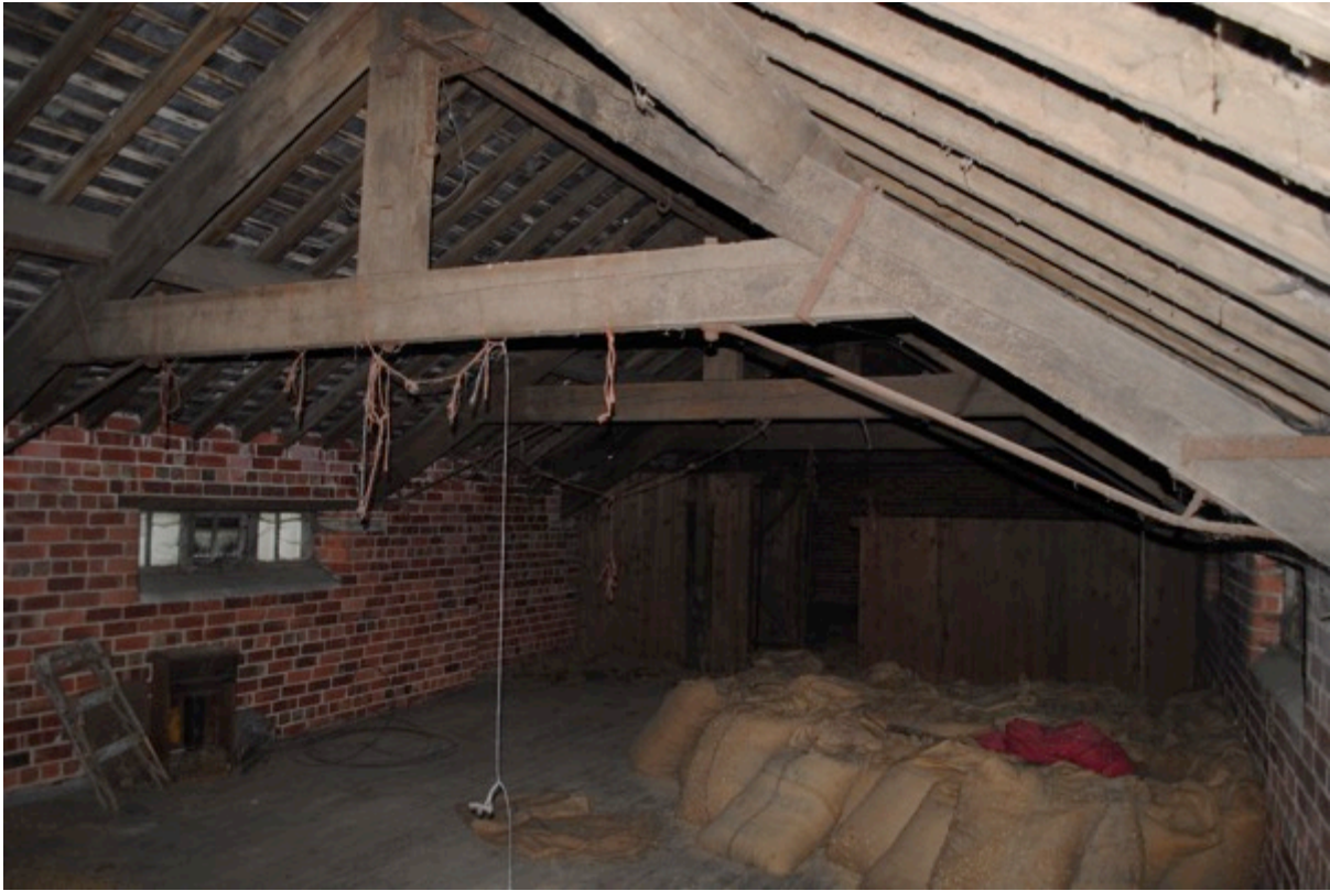
Plate 7: Plot 1, internal second floor, as viewed looking east.
