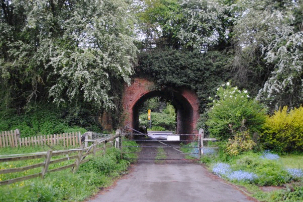
Plate 1: Entrance, beneath the former Bestwood Colliery Branch line, to the study site, as viewed looking west.
