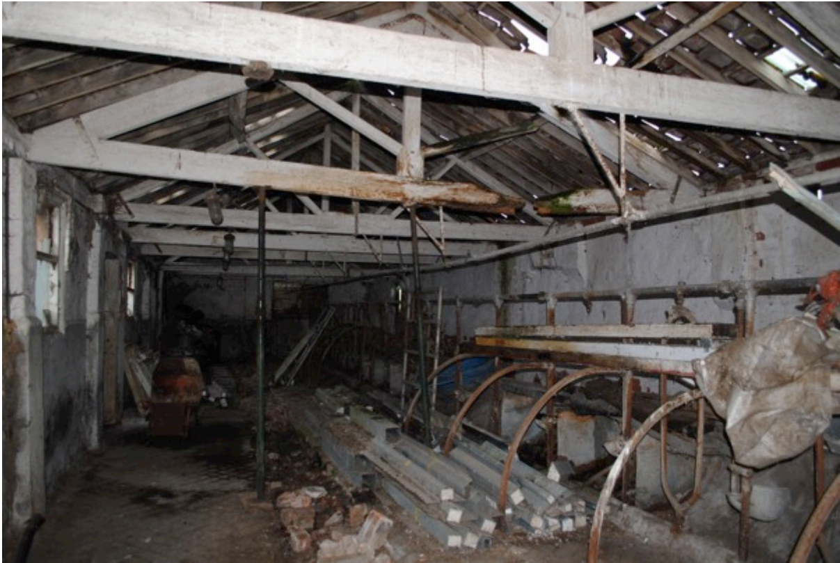
Plate 13: Plot 3, internal, as viewed looking north.
