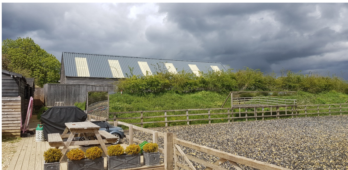
01 – Neighbouring shed in background, bund to be removed
