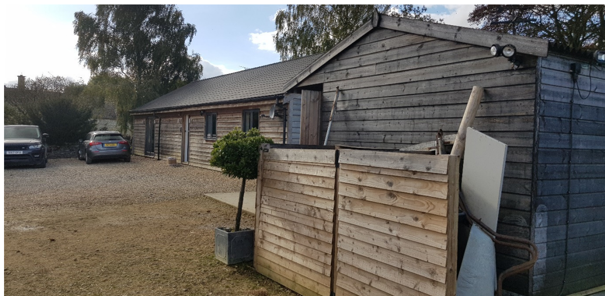
09 – View towards house across yard
