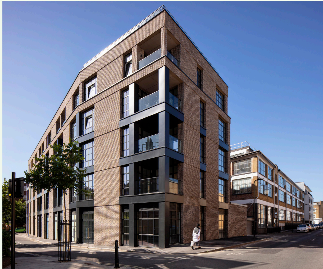
DETAIL FACADE VIEW - EAGLE WHARD ROAD, ISLINGTON (BGY)
