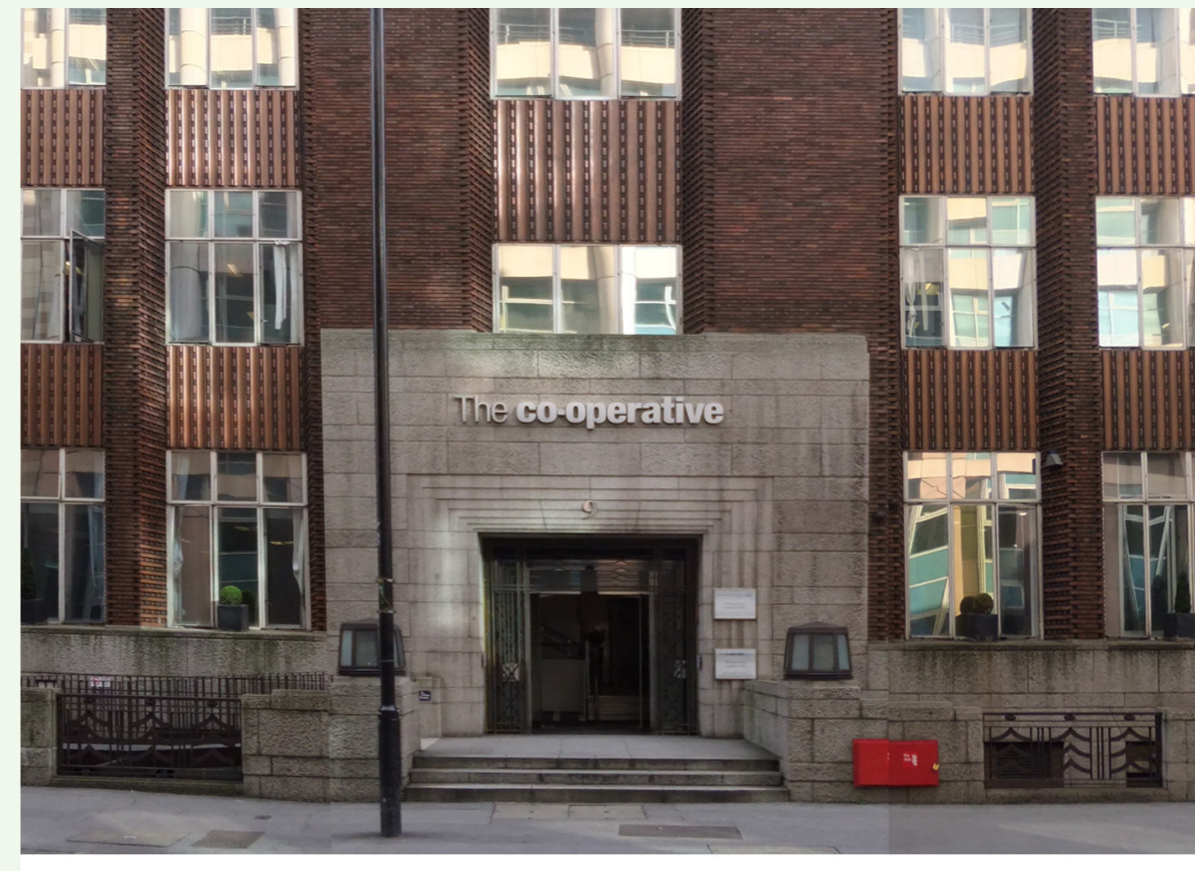
EXISTING PRESCOT STREET BUILDING ENTRANCE
