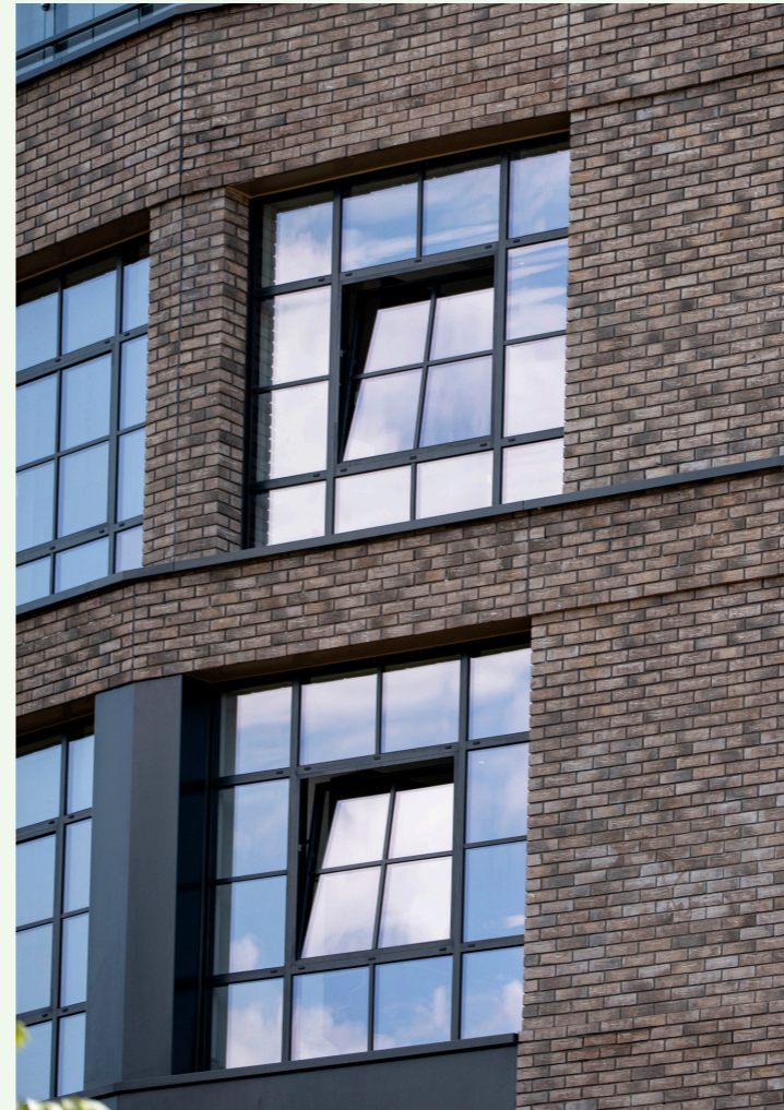
DETAIL FACADE VIEW - EAGLE WHARD ROAD, ISLINGTON (BGY)
