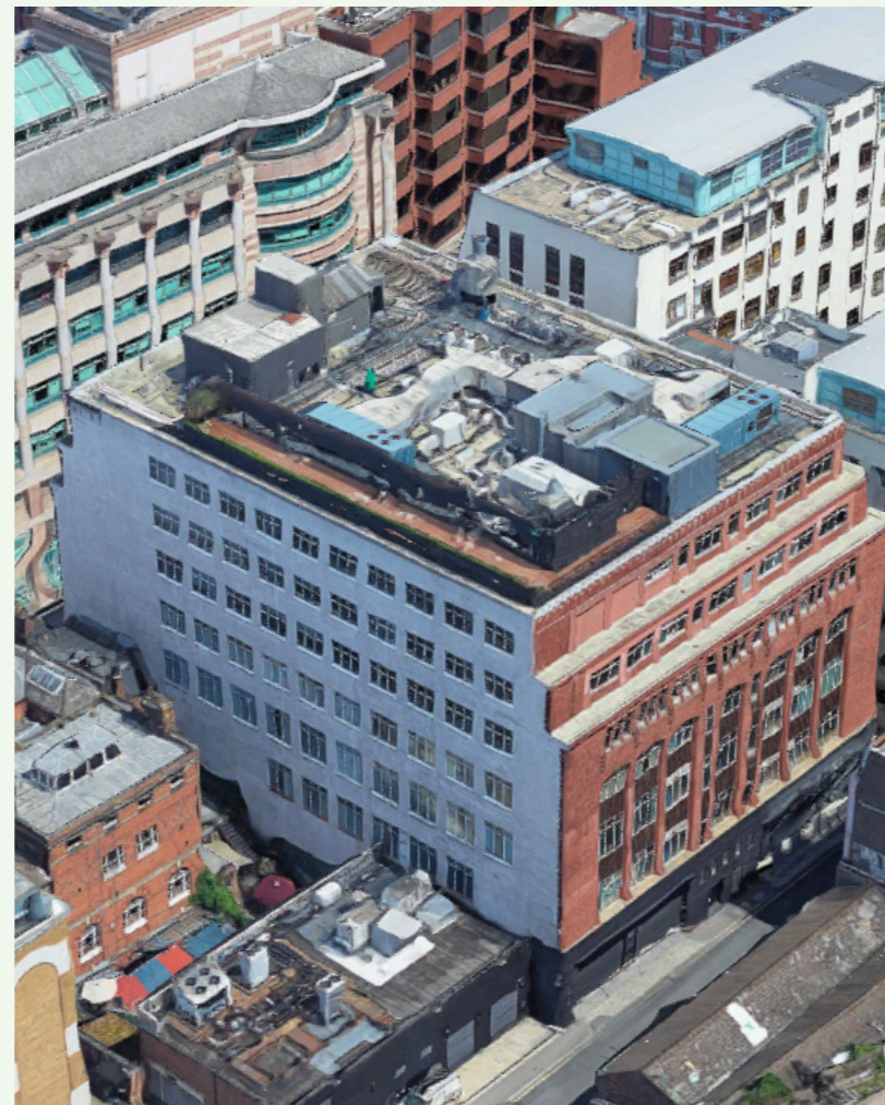
EXISTING WEST GABLE FACADE
