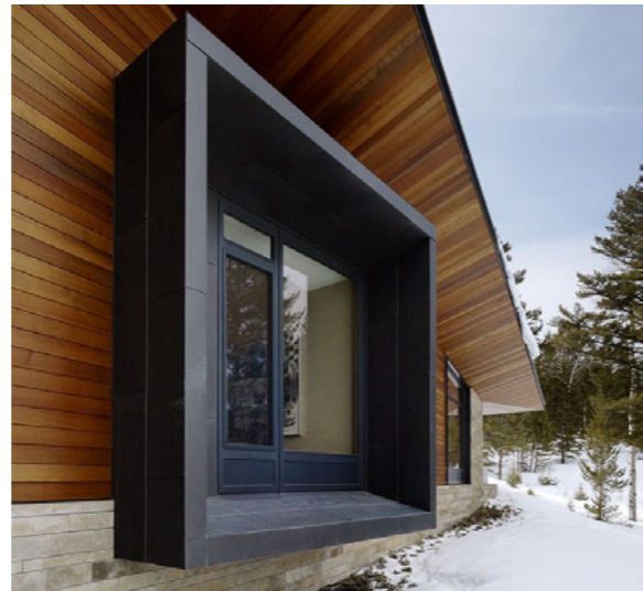
4 Zinc clad protruding window frame
