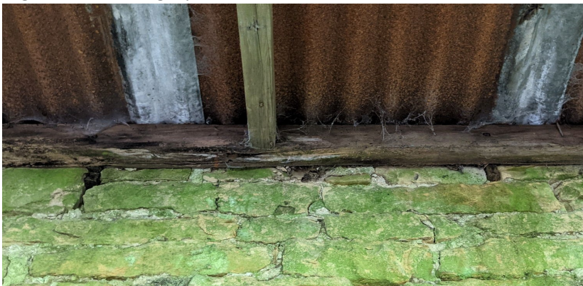
Fig. 1 Timber wedges for external timber attachment:
