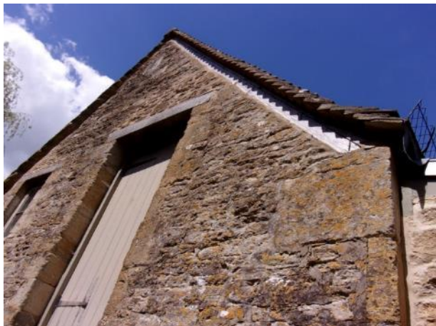
Plate 3.10: Well-sealed gable verges
