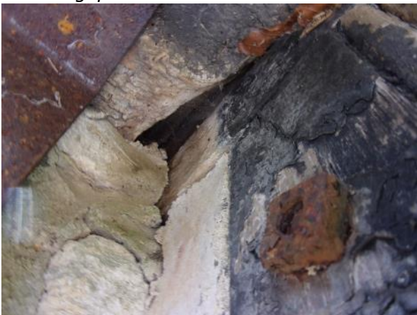
Plate 3.9: Gaps around ground floor door on south elevation
