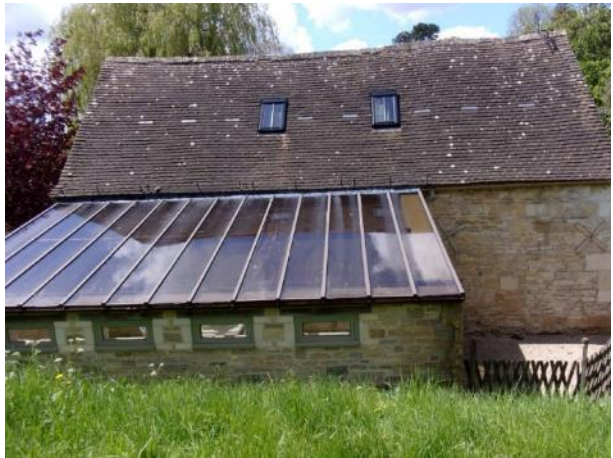
Plate 3.4: East elevation, with concrete-tiled roof pitch and glass-roofed lean-to extension
