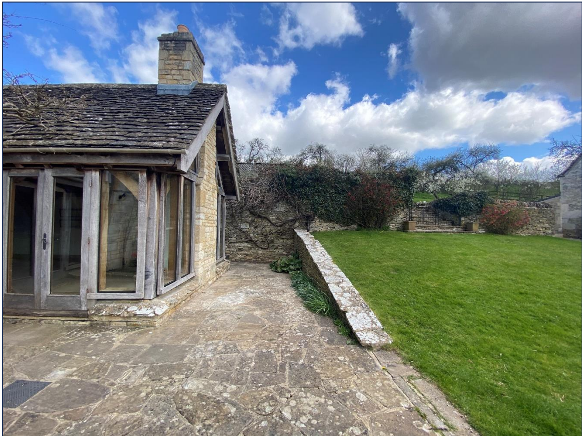
Figure 8: Existing chimney stack
