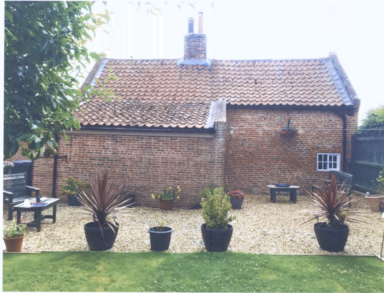
EXISTING VIEW OF REAR OF COTTAGE (NORTH-WEST ELEVATION)
