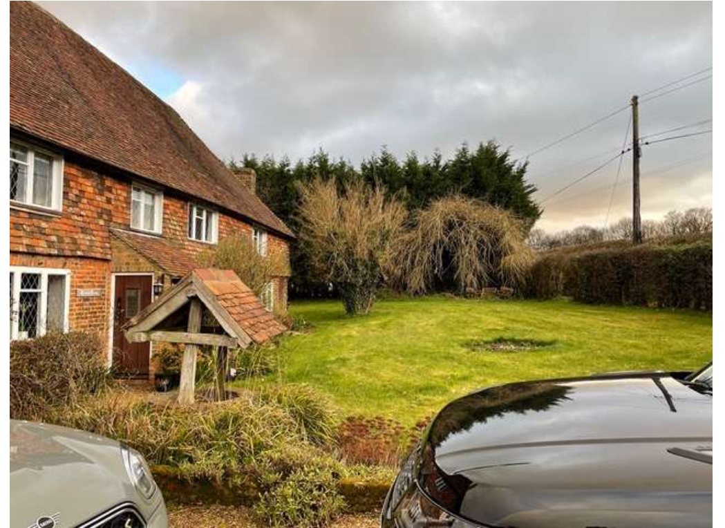
North West elevation of the porch entrance
