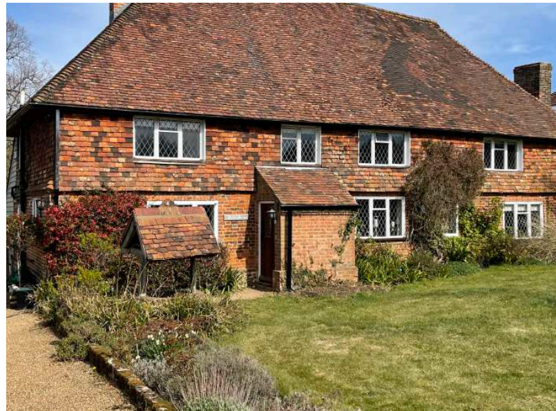
View of Access from the North West
