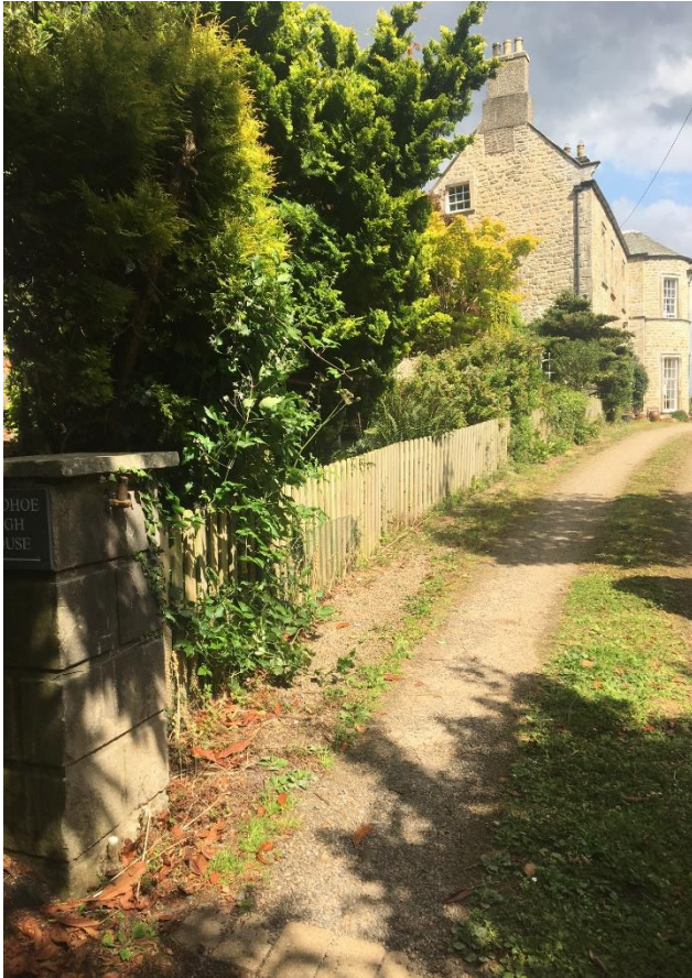
SANDHOE HIGH HOUSE – existing timber fence to front (primary) elevation
