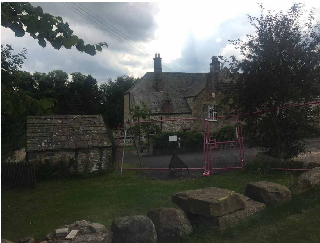
SANDHOE HIGH HOUSE – rear elevation in far background
