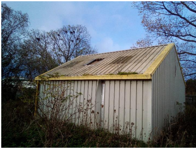
Photo 11. Building 11 – Pump house
