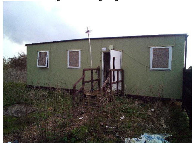
Photo 4. Building 4 – Portable cabin
