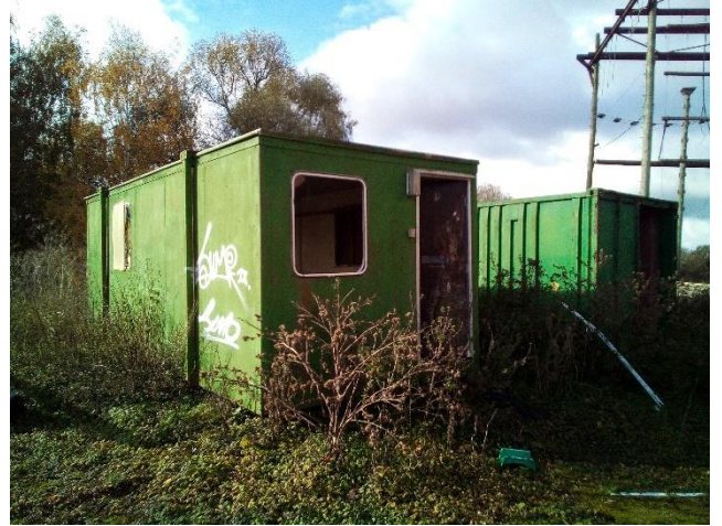
Photo 8. Building 8 -Portable cabin
