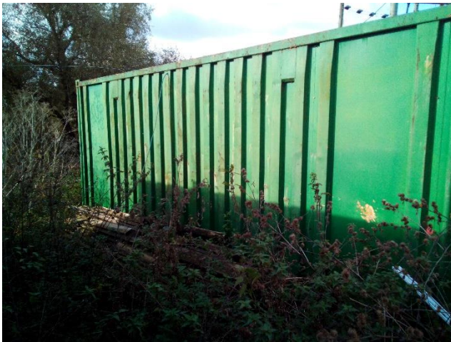
Photo 9. Building 9 – Shipping container
