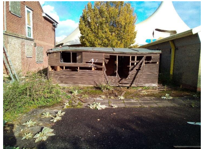
Photo 12. Building 12 – Wooden shed
