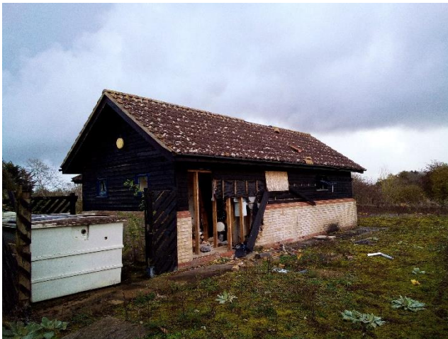
Photo 3. Building 3 – Toilet block
