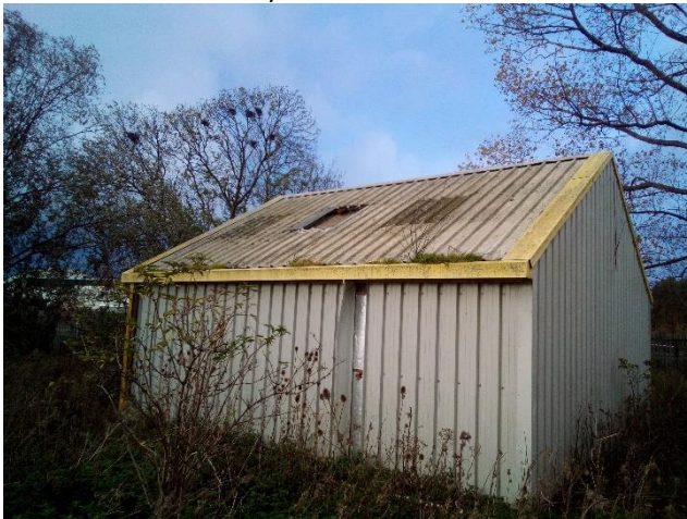
Photo 36. B11 – Pump house
