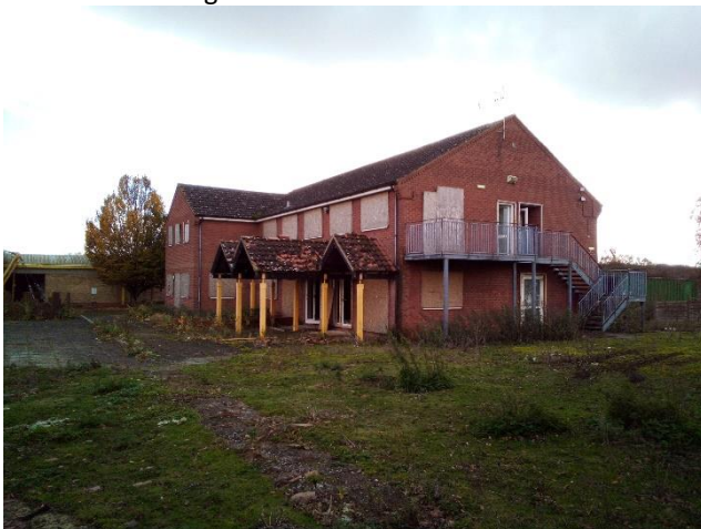
Photo 5. Building 5 – Residential property
