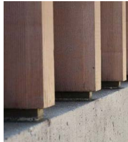
timber cladding on concrete upstand
