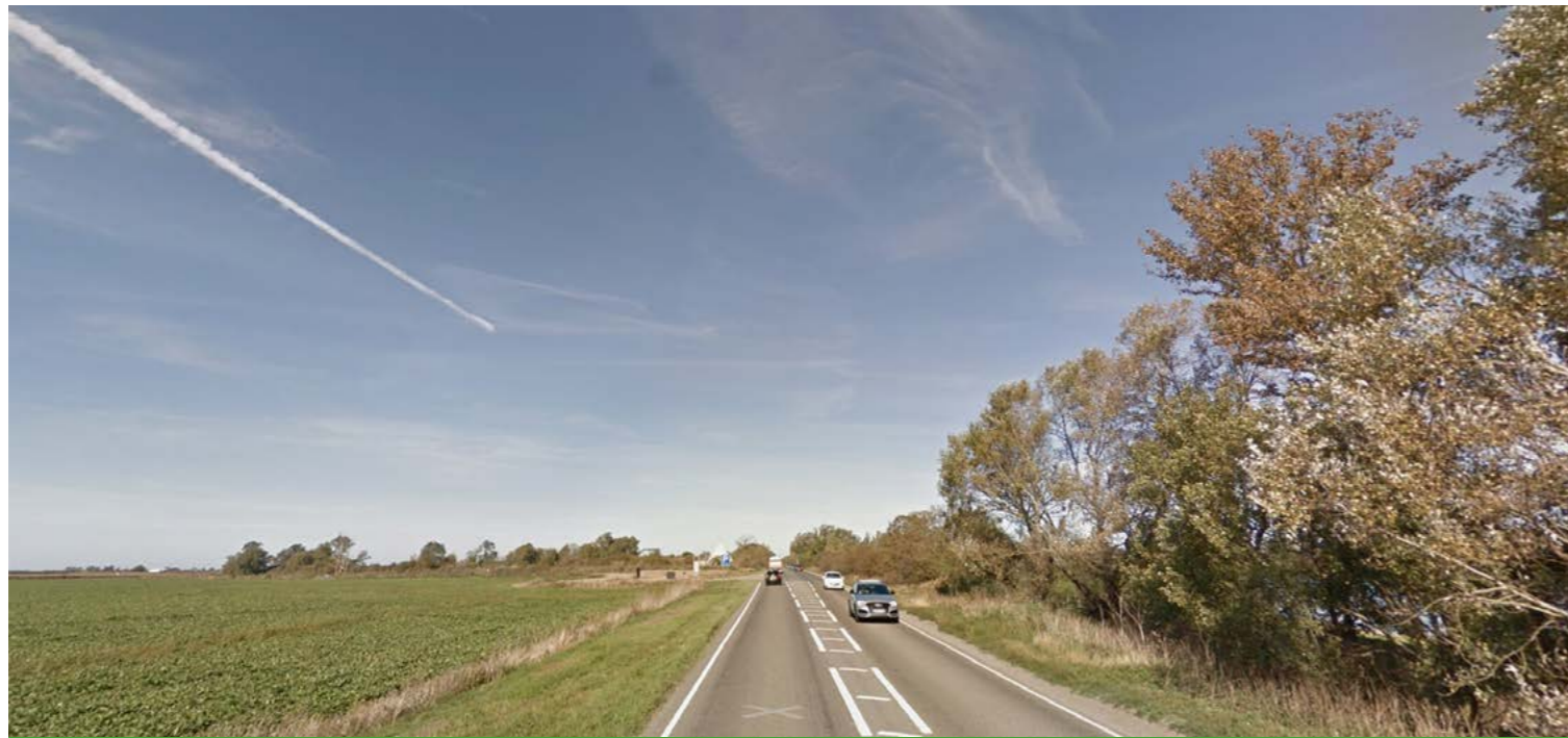
view looking north on A412 with site on the left in the distance
