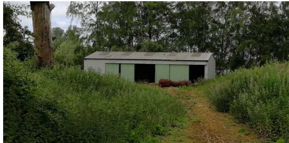
Existing structure to be replaced
