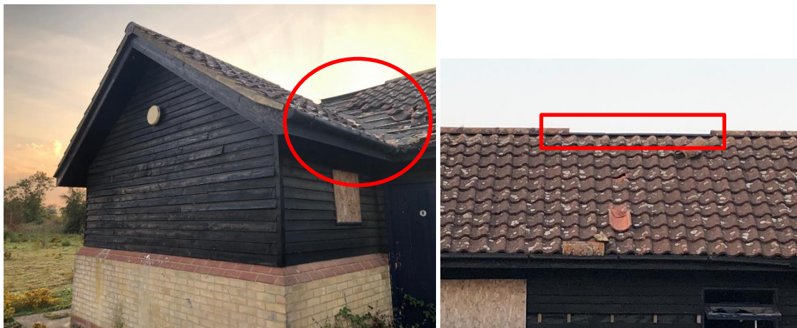
Example of tiles removed from roof
