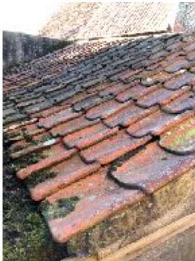
View of original roof space
