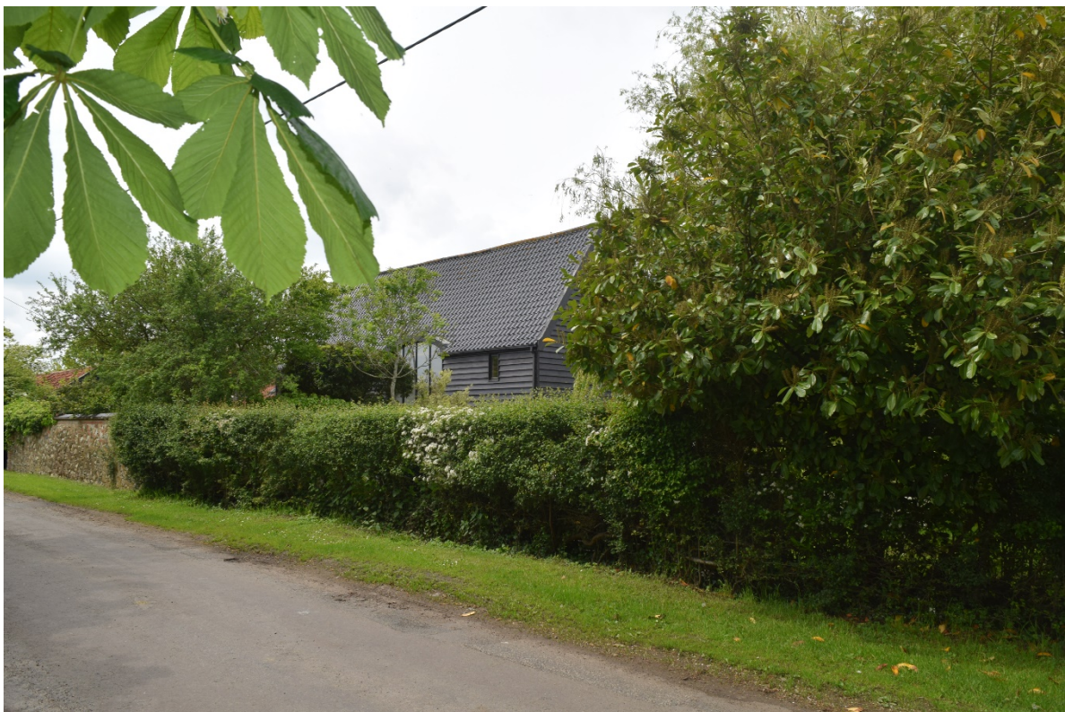
Figure 8: Sudbourne Farm Barn - View of Sudbourne Farm Barn's frontage to Mill Road.
