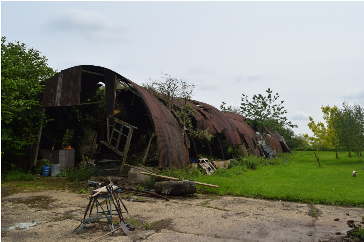
Figure 15: Existing Nissen Hut on the proposed development site.
