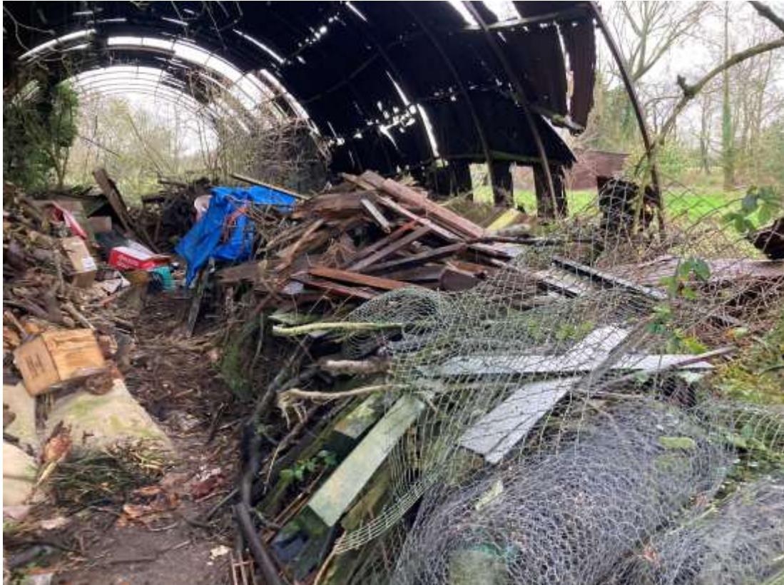
Photograph 2: Inside of Nissan Hut on Land at Forge Barn, Wyverstone.
