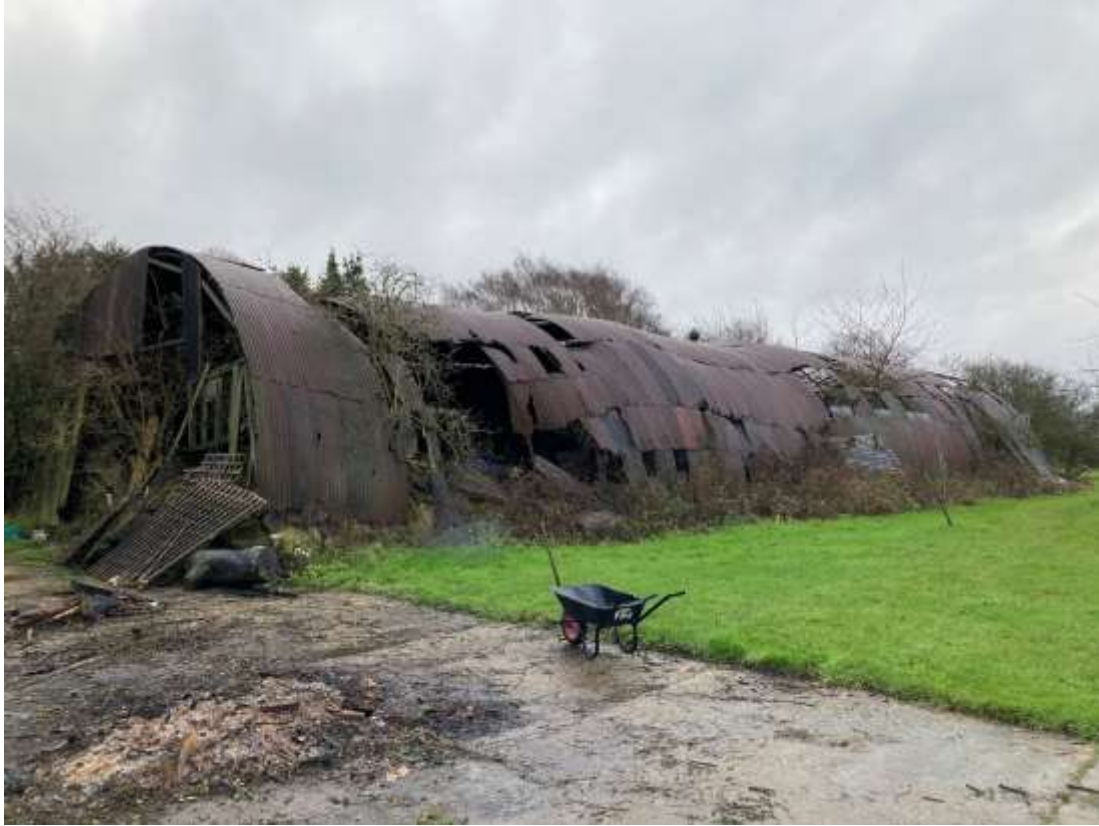
Photograph 1: Nissan Hut on Land at Forge Barn, Wyverstone.
