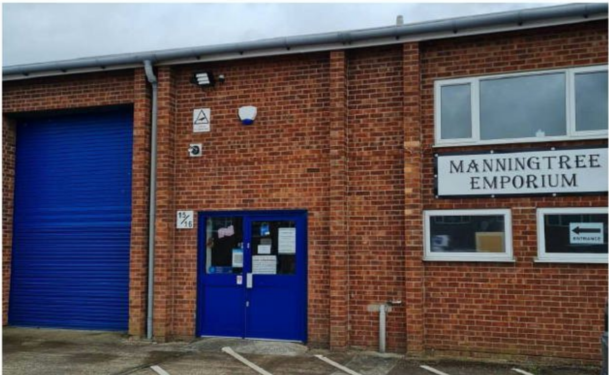
Fig. 2 – Front view of 15-16 from the car park
