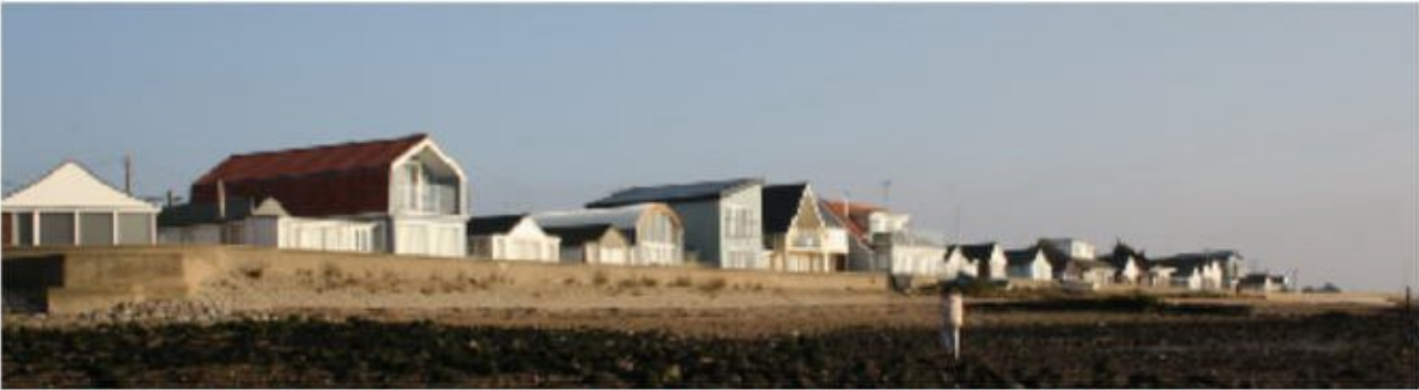
Fig 8: Photograph demonstrating the pattern of original short chalets and the newly build chalets all set behind the seawall.
