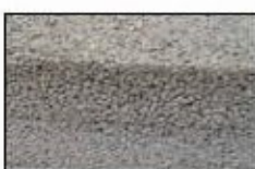
Concrete finish chosen for sustainability and some SUDS drainage
