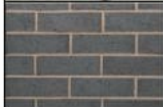
Blue/Grey Engineering Brick Lower Ground Floor
