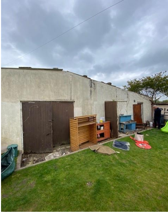
Front Elevation from Rear Garden of main dwelling.
