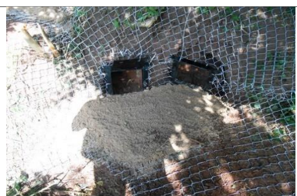
Plate 4: Once the gates are secure sand traps should be installed outside and inside the gate to monitor badger activity.
