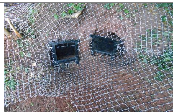
Plate 3: Holes are then cut in the fencing over each hole and the gates are secured into the chainlink using the metal cable ties.
