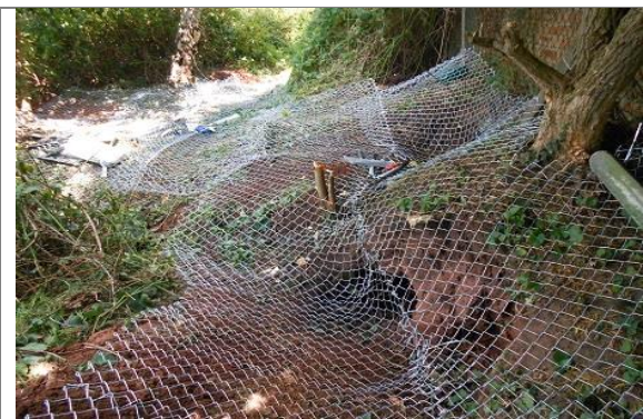
Plate 1: The area surrounding and including all Sett entrances are to be covered In Chainlink Fence. The fencing is then to be pinned to the ground using the 1" posts.
