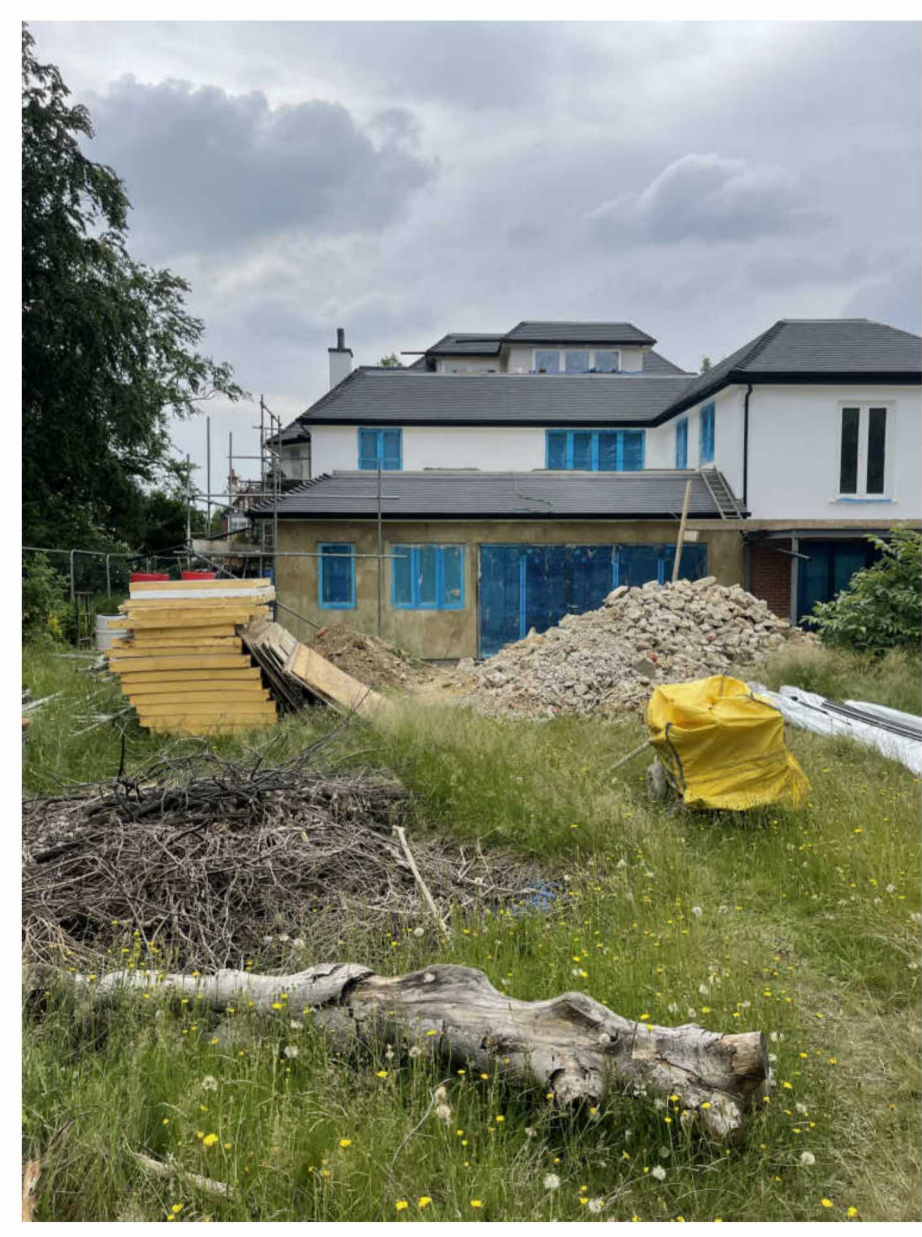
As-built rear dormers
