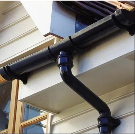
Black cast iron rainwater goods
