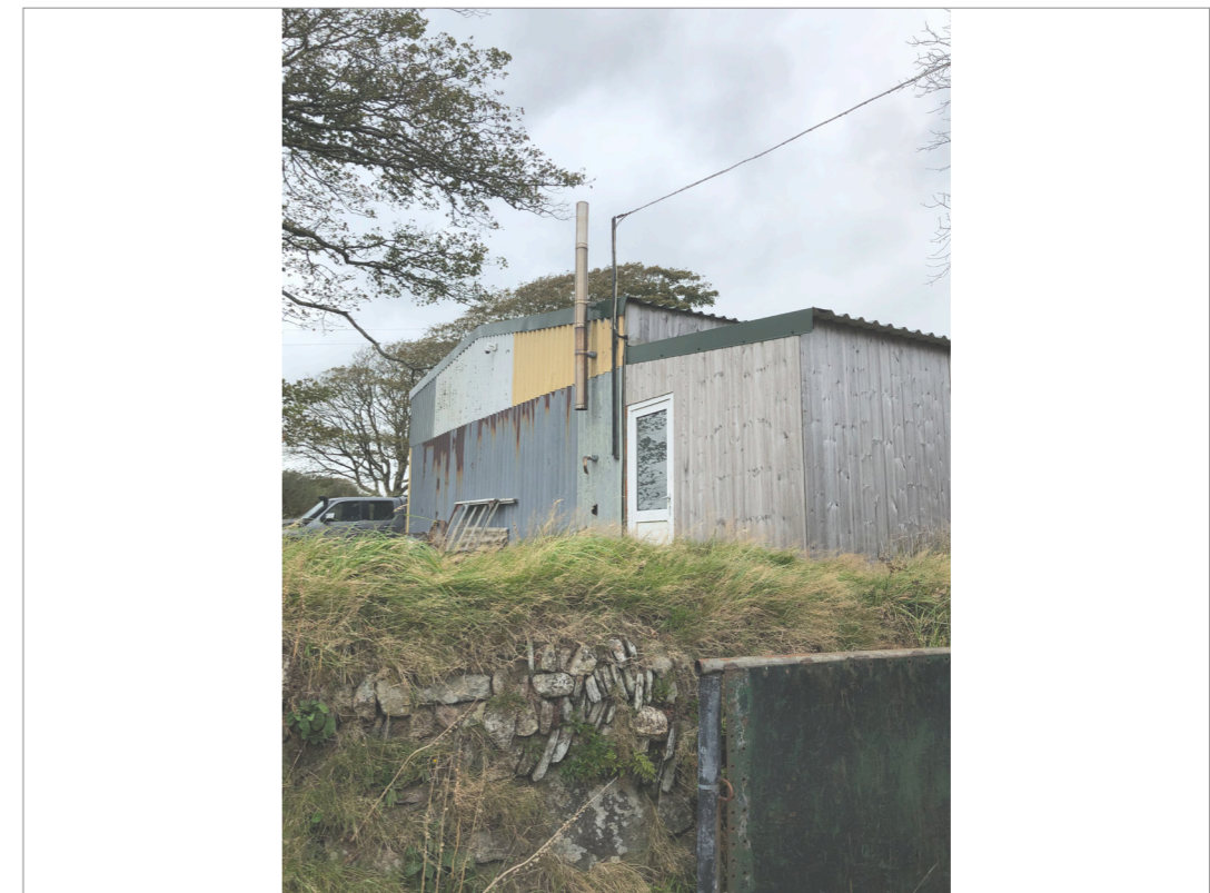
VIEW OF EXISTING OLD WORKSHOP
