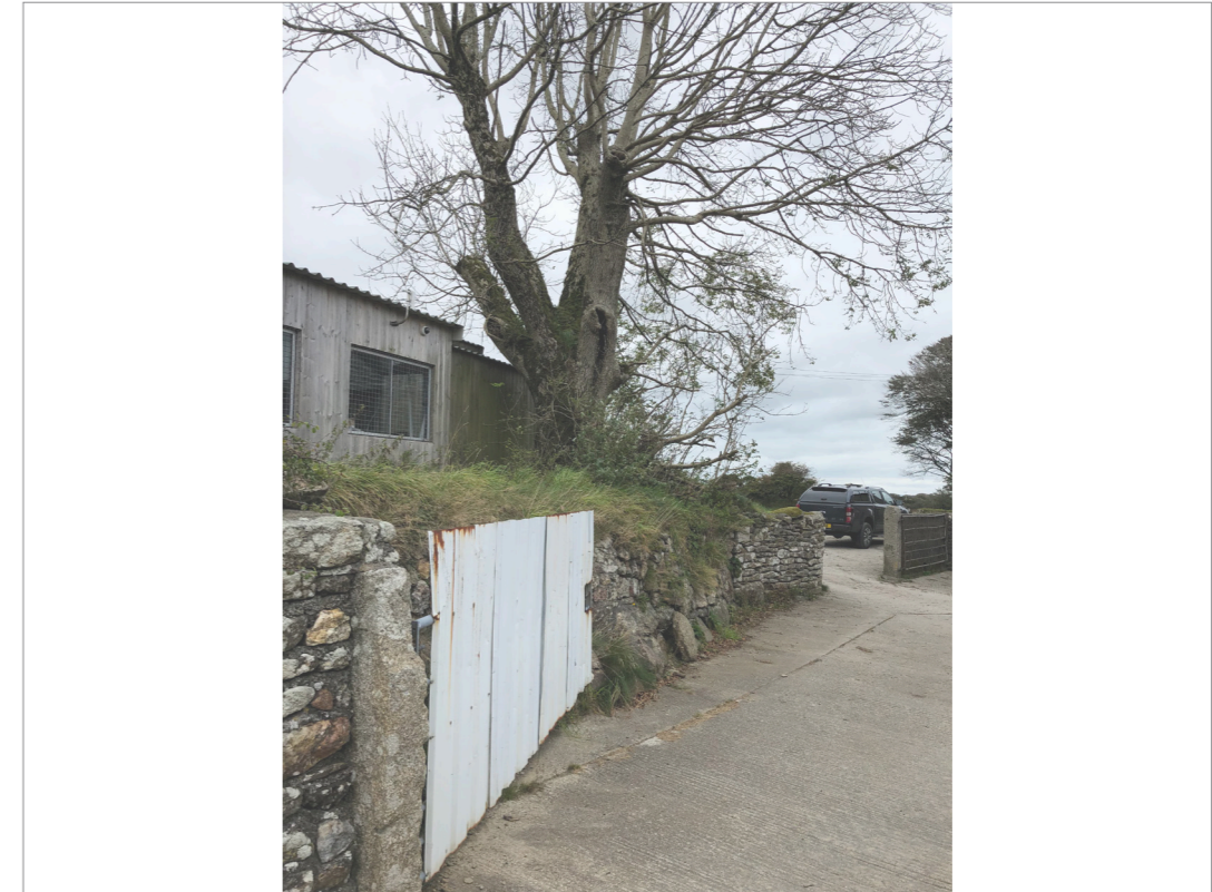
VIEW OF EXISTING OLD WORKSHOP
