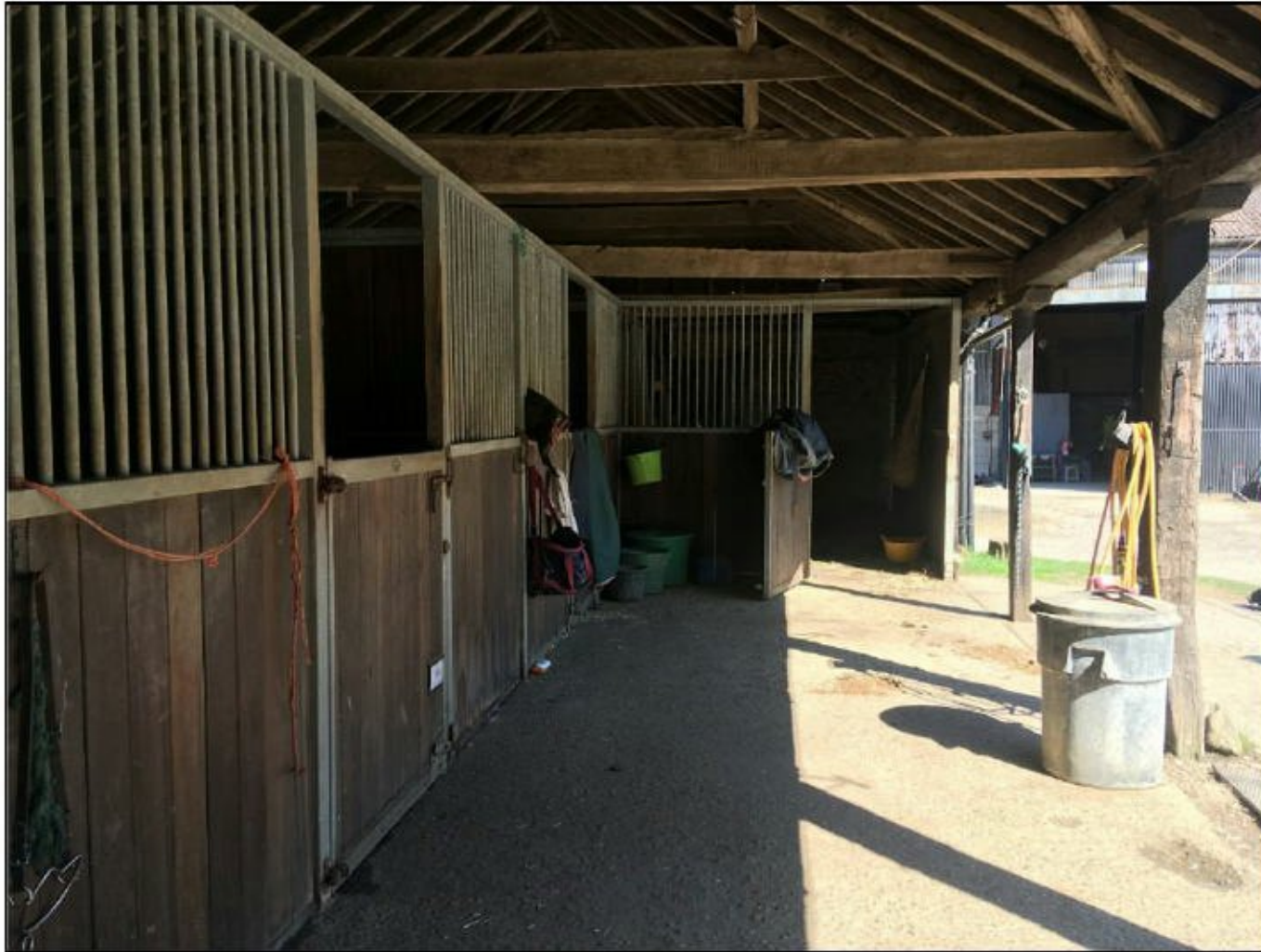
Photograph 3: The cartlodge in use as stables.
