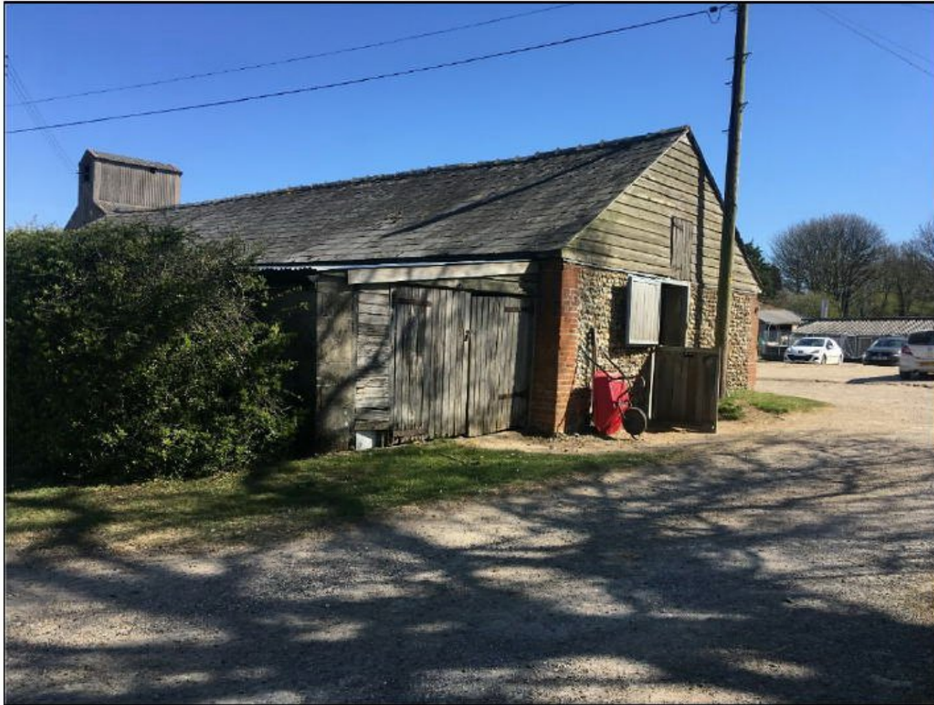
Photograph 9: The southern side of the cartlodge with the extension in use for storage and an additional stable.
