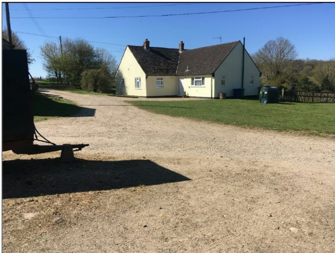
Photograph 14: The bungalow to the west of the site.
