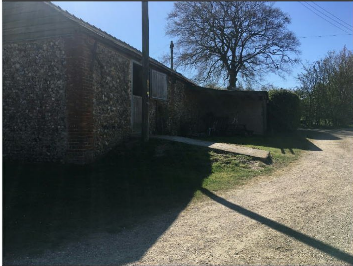
Photograph 5: The western sector of the site with an additional stable fronted by a concrete ramp.
