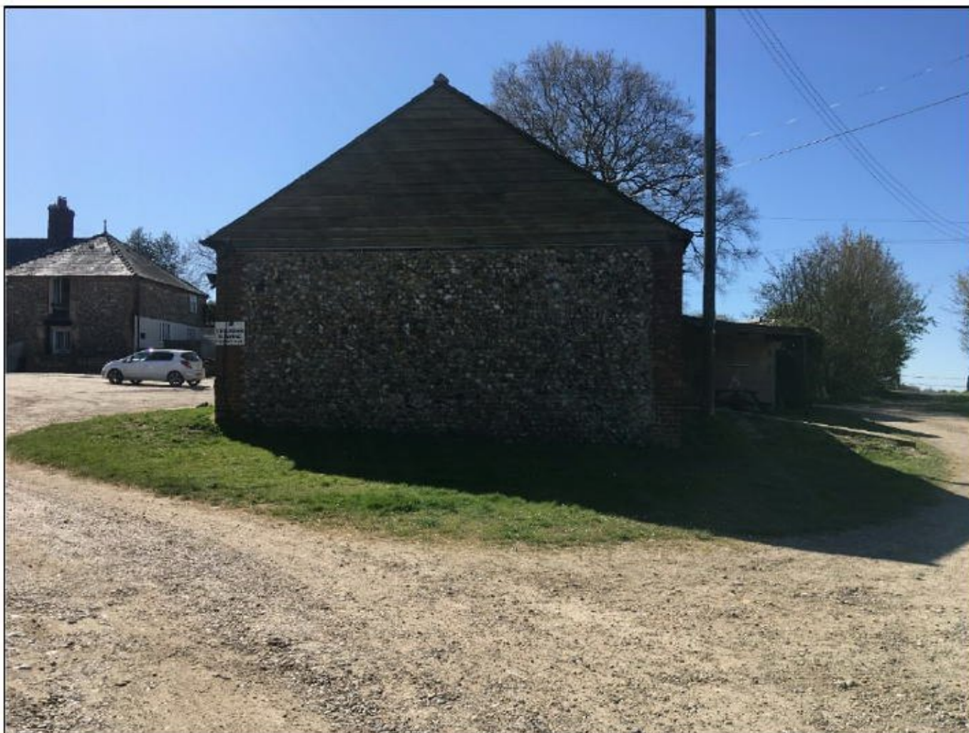
Photograph 4: The northern wall of the cartlodge.
