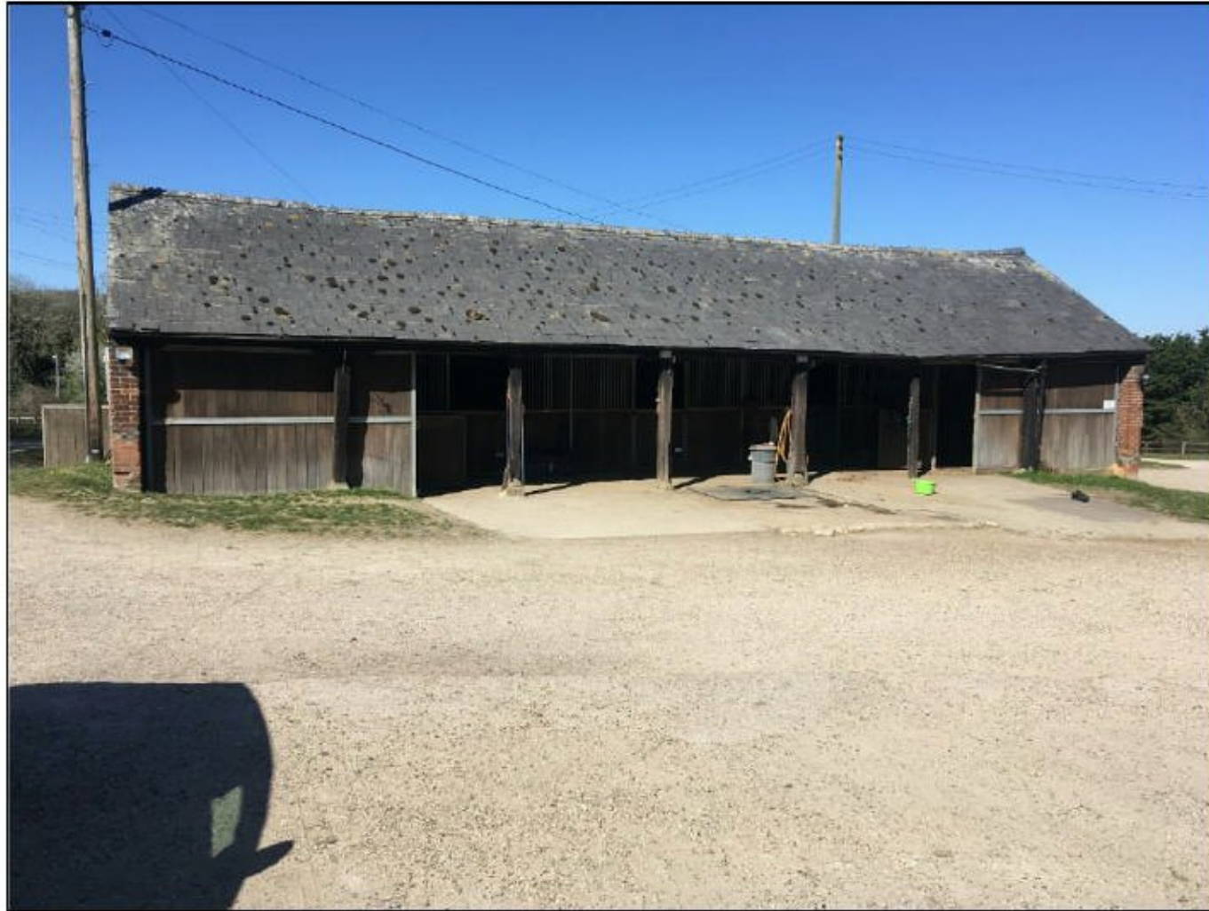
Photograph 1: The cartlodge from the east.
