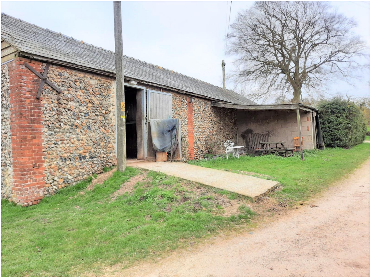
Rear (West facing) elevation
