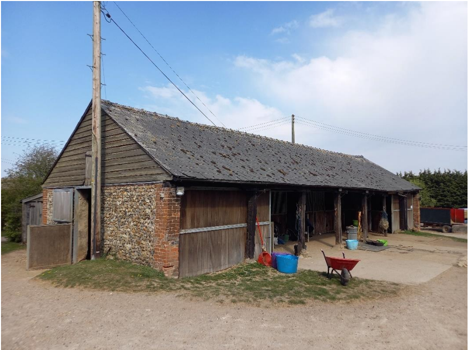
Plate 4.1.1: Southern and eastern elevations
