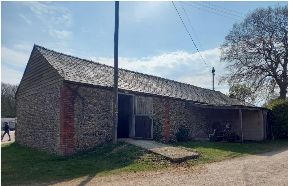
Plate 4.1.2: Northern and western elevations
