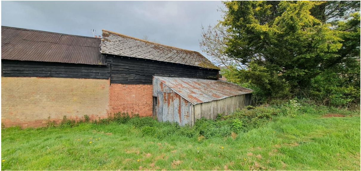
PHOTO PAGE 4 – EASTERN FACE OF BARN
