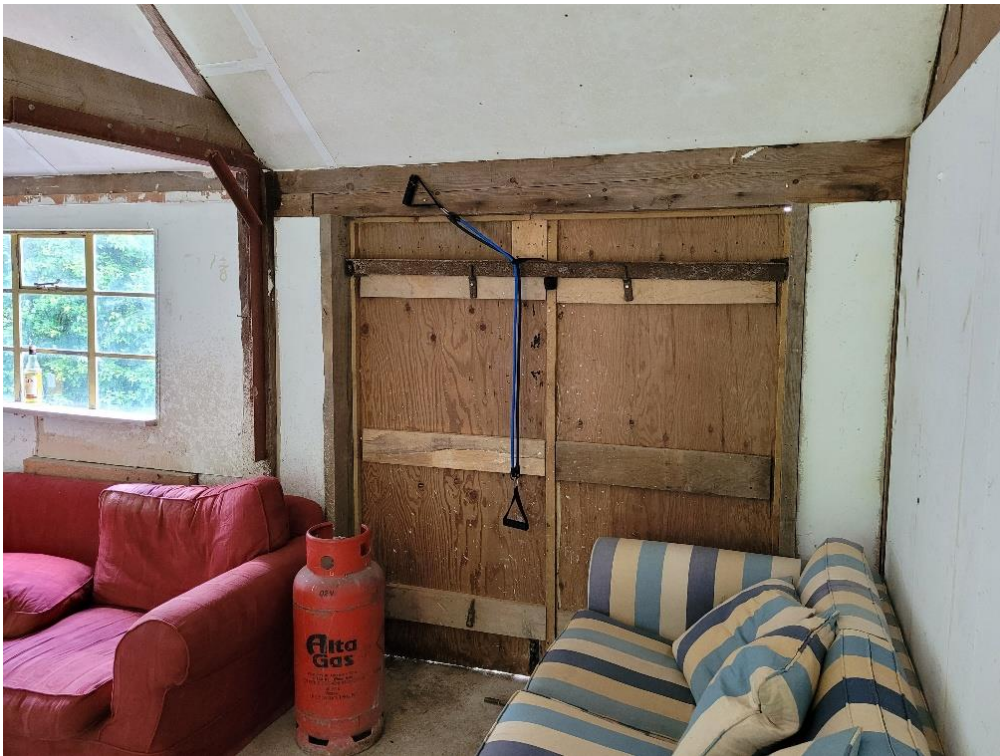
Interior looking north
