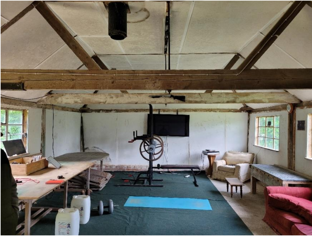
Interior looking west
