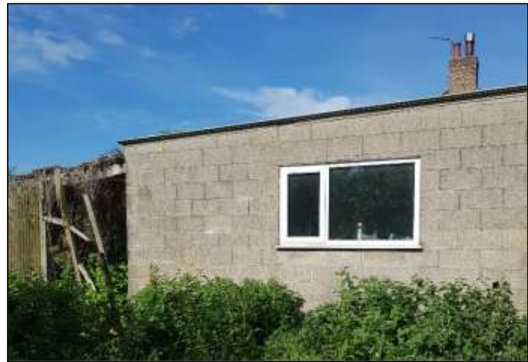
Image 5: Views of buildings to be demolished.
