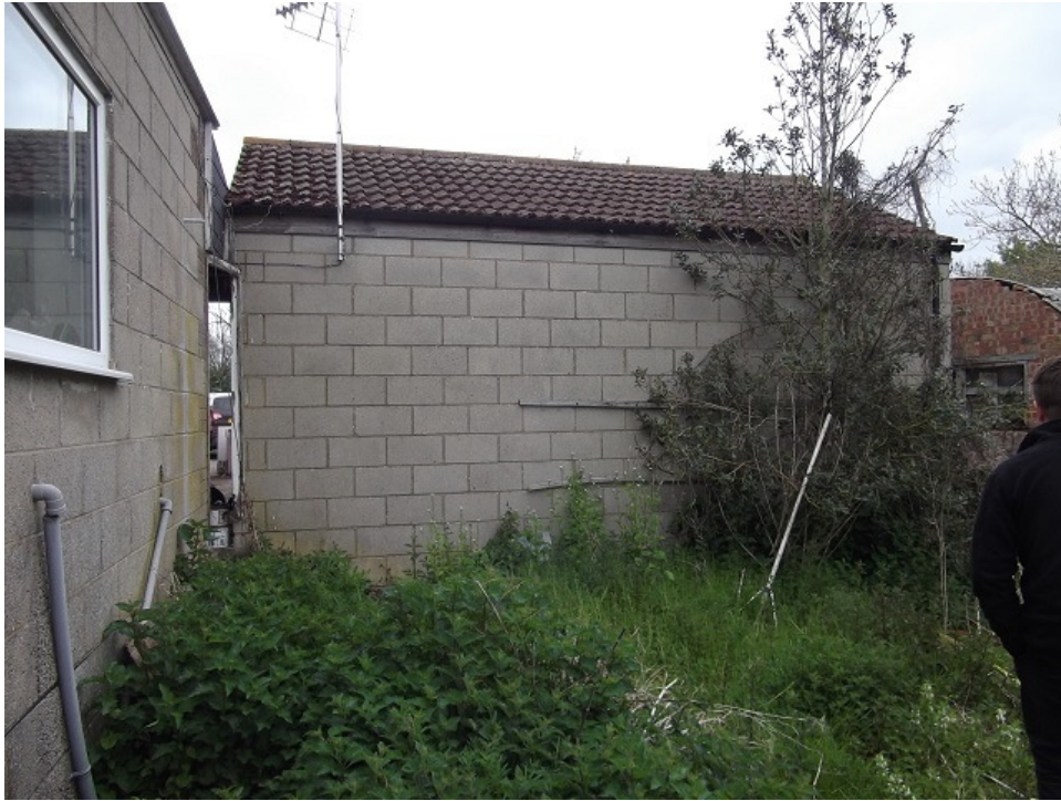
Plate 10. The south elevation of Buildings 2.
