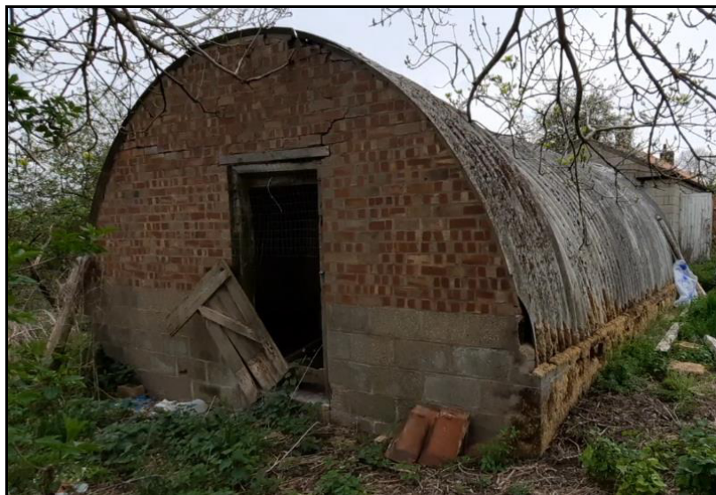
Plates 2a to c – Building 1 eastern gable with gap above the door frame, and the interior of the building.
