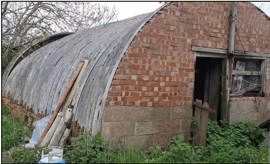
Plates 2a to c – Building 1 eastern gable with gap above the door frame, and the interior of the building.
