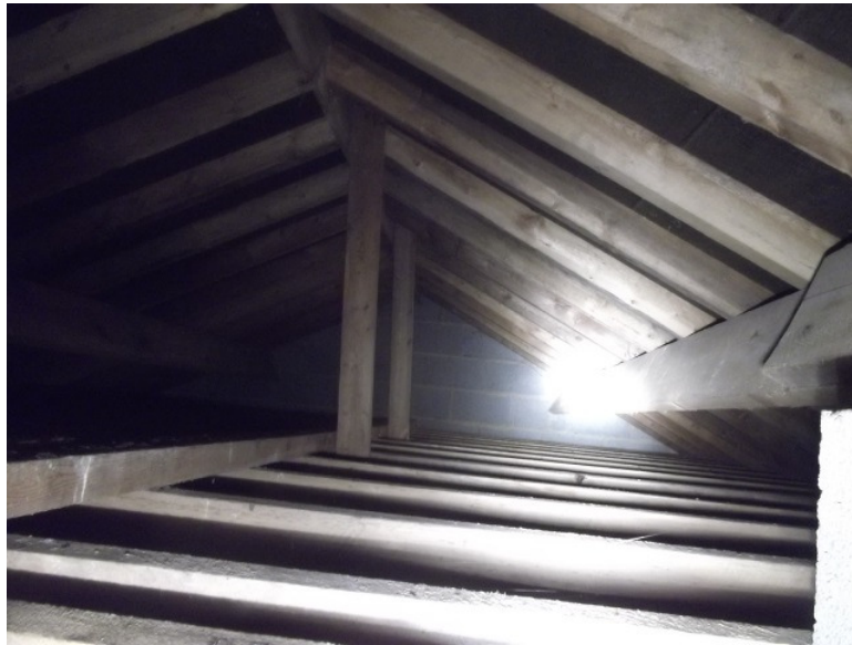
Plate 6 – Building 2 pipe hole allows access into the block wall cavity
