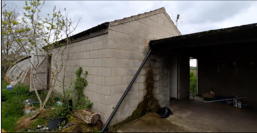
Photo 9 - The adjoining cladding for the carport is not pointed (screw fixed) with gaps to the under and connecting sides.
