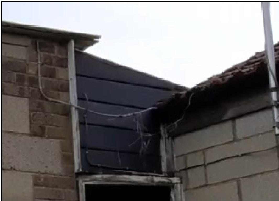
Photo 9 - The adjoining cladding for the carport is not pointed (screw fixed) with gaps to the under and connecting sides.
