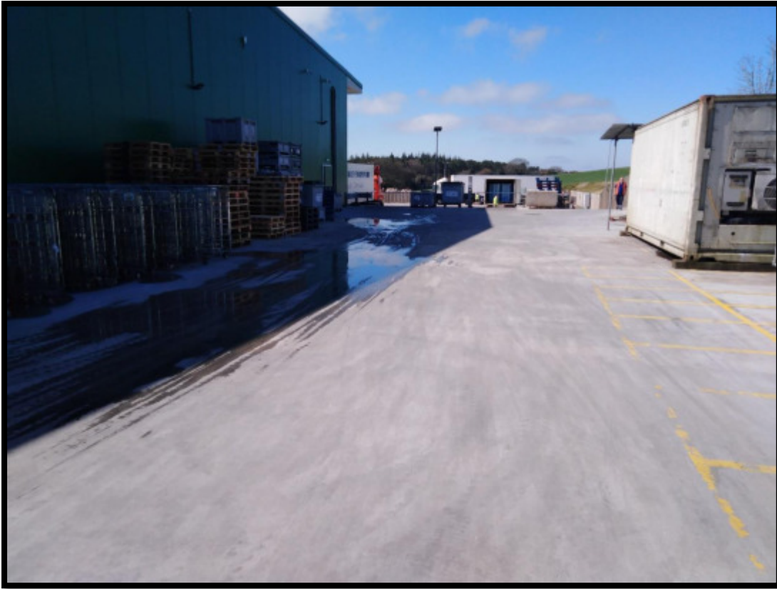
Photograph 1 – Area 1: Southern half, view from east, looking west.
