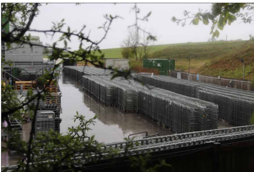
Plate 3: The site of the proposed refrigerated loading bay extension, looking northwest. The extent of terracing for the existing infrastructure is clearly visible
