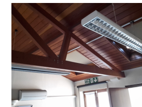
Existing Timber Truss
