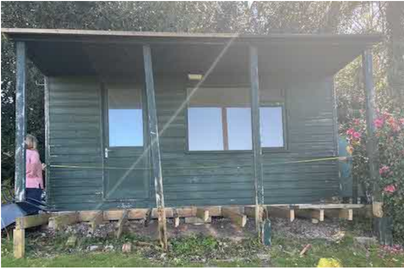
Previous arrangement, show with deck partially dismantled
